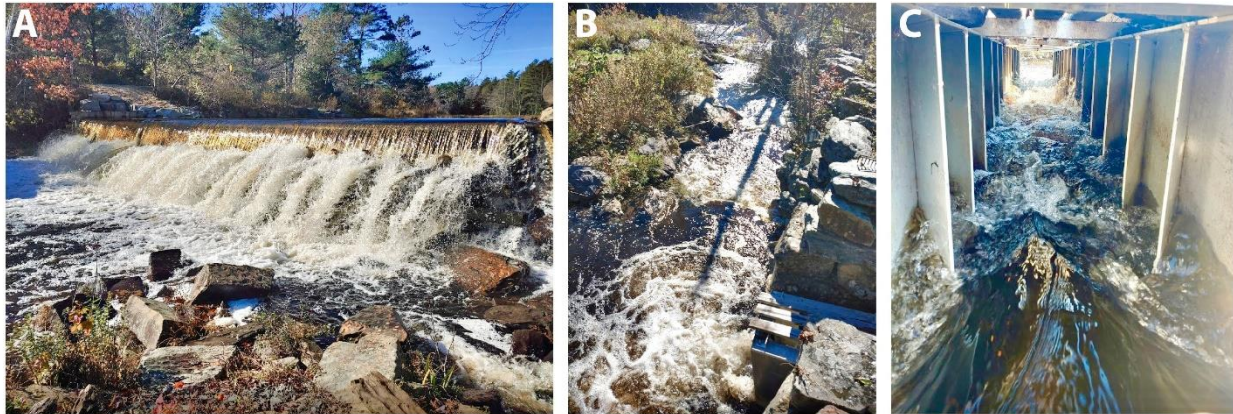
Figure A1. Crousetown Dam (A) showing stepped pools (B) and inside of Denil ladder (C).
