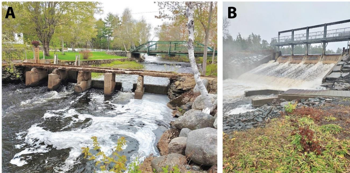
Figure A2. Cranberry Dam (A) and Hebb Dam (B) showing base of fish ladder.
