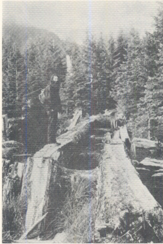
Figure 6: Remains of the 'fore-and-aft' main logging road from the mouth of Mathers Creek to Mathers Lake.
