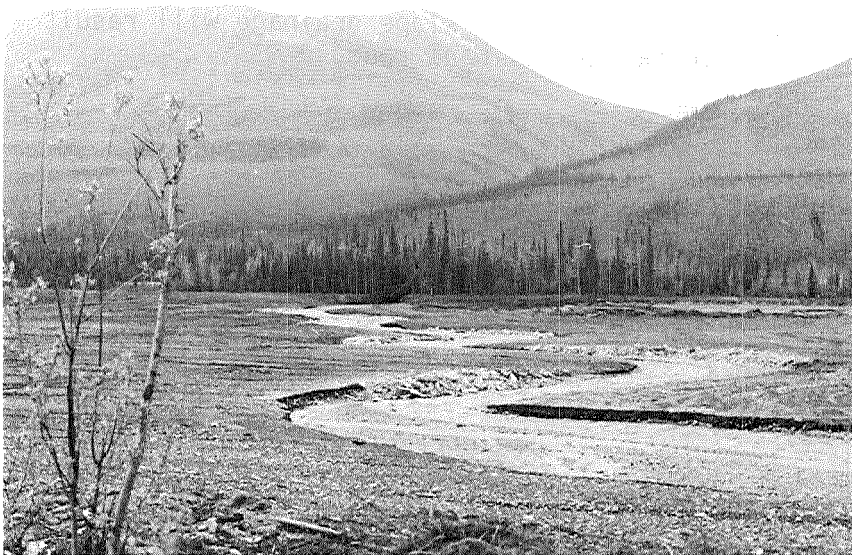
Fig. 24. Rehabilitated materials site, Brooks Range area. Note rechanneled stream and bank stabilization. Area is to be revegetated.
