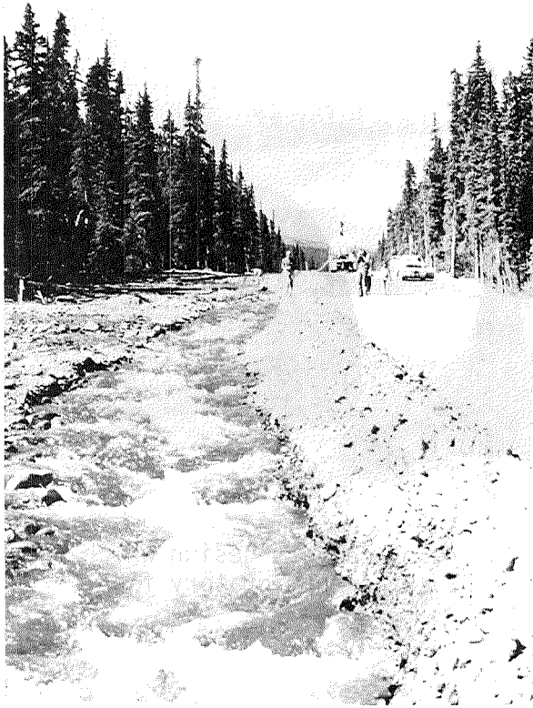
Fig. 18. Improper alignment of pipeline resulting in flow of glacial meltwater along right-of-way and the deposit of silt in an important salmon and nursery area on the Little Tonsina River.
