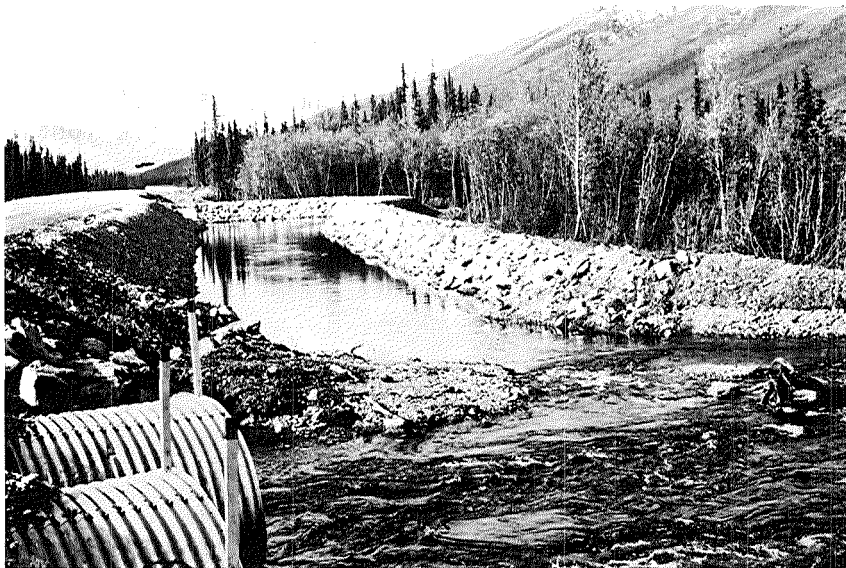
Fig. 21. Marion Creek culverts and fishway.
