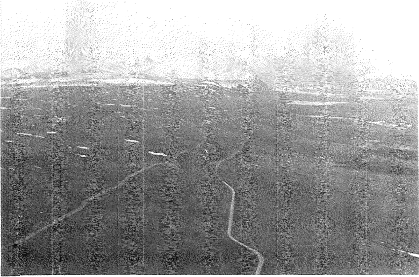
Fig. 7. Zigzag configuration of above-ground selection of pipeline (left) and haul road, Yukon River area.
