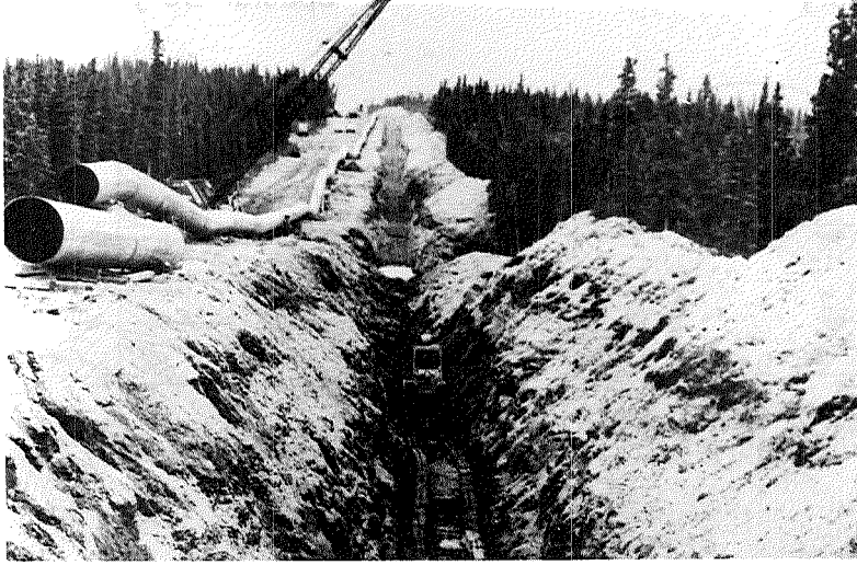
Fig. 5. Preparation of trench for buried segment of the pipeline.
