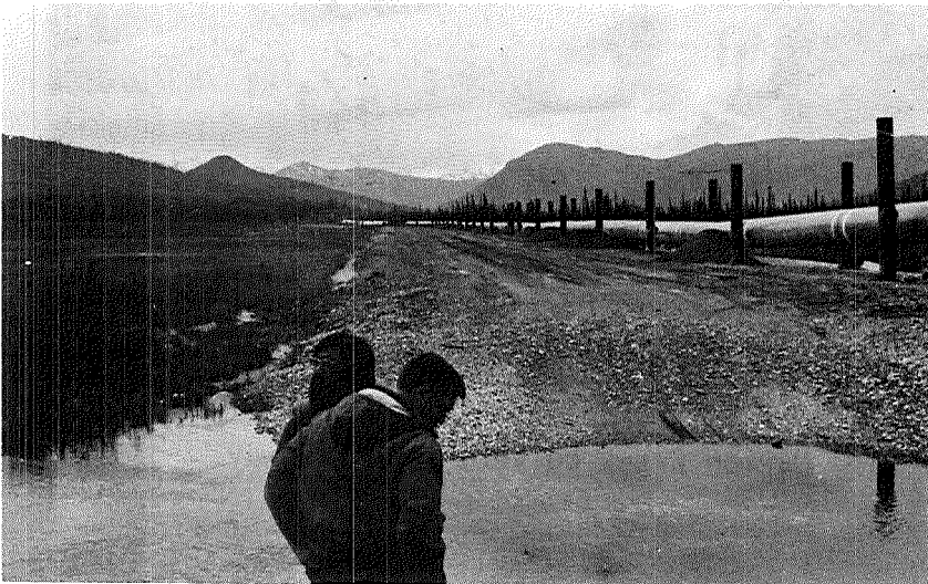
Fig. 19. Low-water-crossing of small grayling stream, Brooks Range area.
