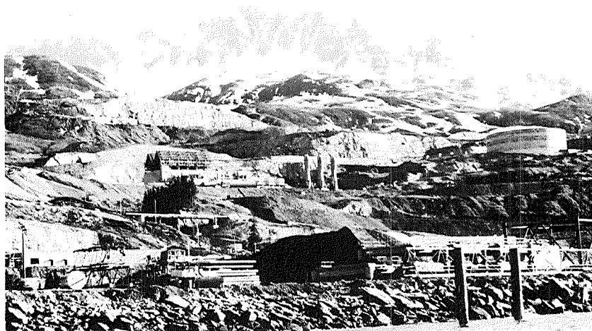
Fig. 13. Construction in progress at Valdez Terminal, June 1976
