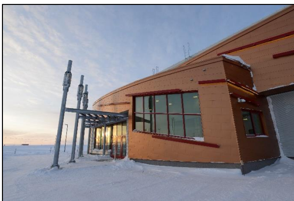
The Canadian High Arctic Research Station Main Research Building
