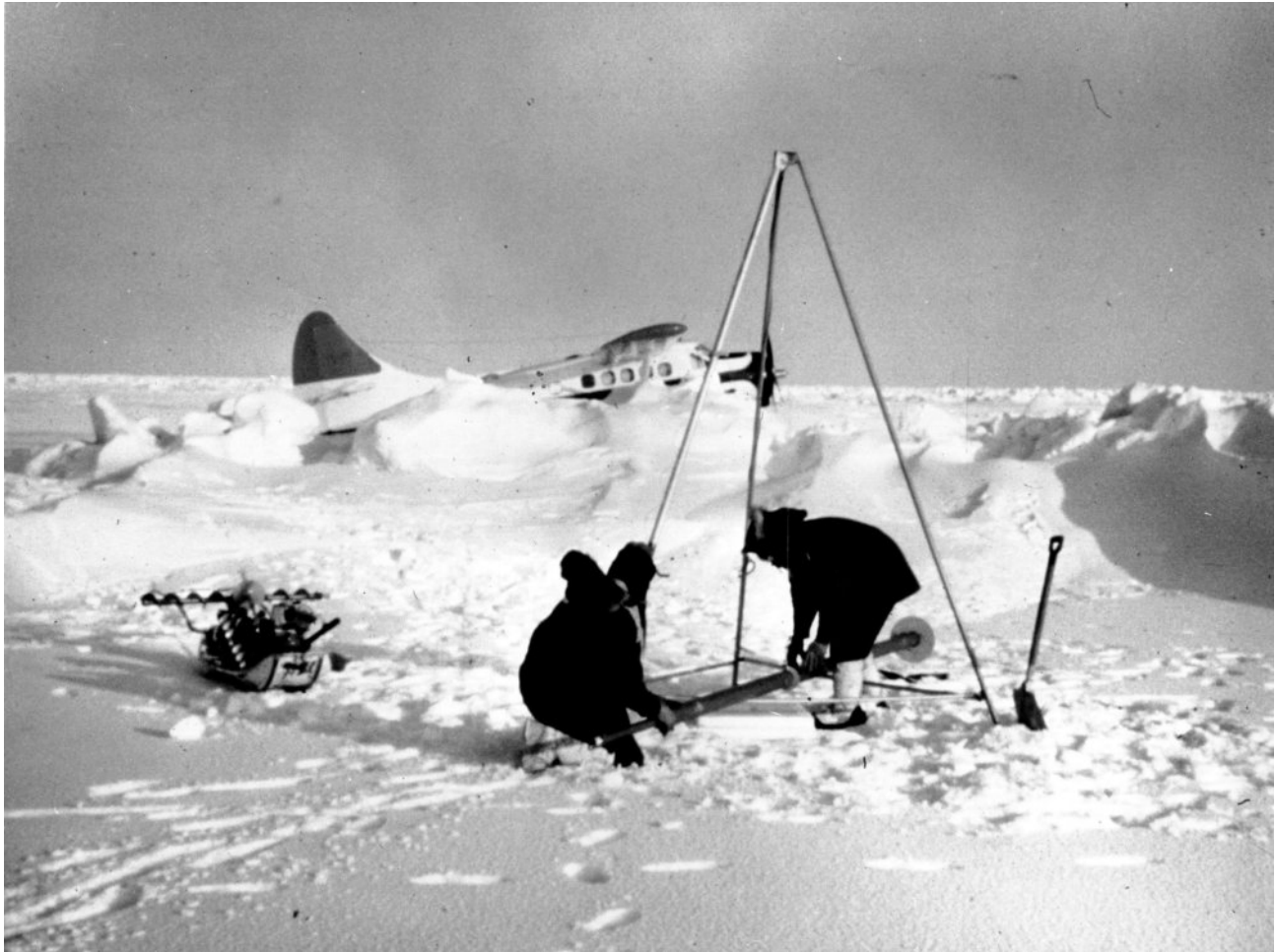
Figure 75: An Ice-Buoy being prepared for installation through the ice. Photo credit: DRDC.
