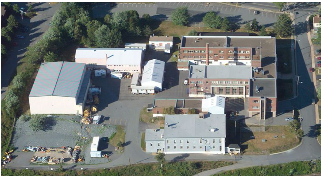
Figure 125: A picture of the former DRDC Atlantic Laboratory. In 1952 the main building was smaller. There have been four extensions added to the original building, and none of the outlying buildings was in existence in 1952 except for the historic “French Cable Building” in the foreground (centre). Photo credit: DRDC.
