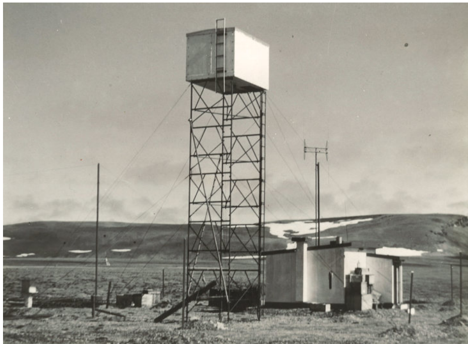
Figure 22: A tower for an auroral spectrograph. The picture was taken in Resolute Bay, looking eastward to the hills on the other side of the runway. The present-day view from this point would be cluttered with buildings. Photo credit: Harold Serson Collection, DRDC – Ottawa Research Centre.
