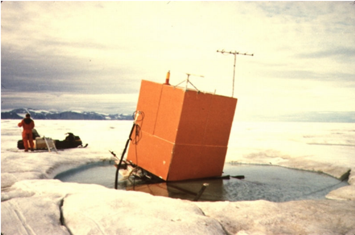
Figure 102: Battery hut after its supporting structure had collapsed. Photo credit: DRDC.
