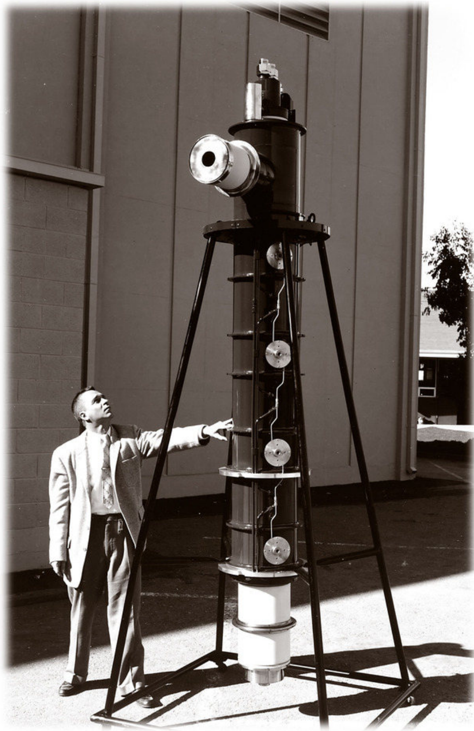
Figure 42: A VA-842 klystron. Klystrons were more powerful and more stable in frequency than magnetrons. Photo taken from Reference [33]. Photo credit: Courtesy of the Silicon Valley Historical Association.
