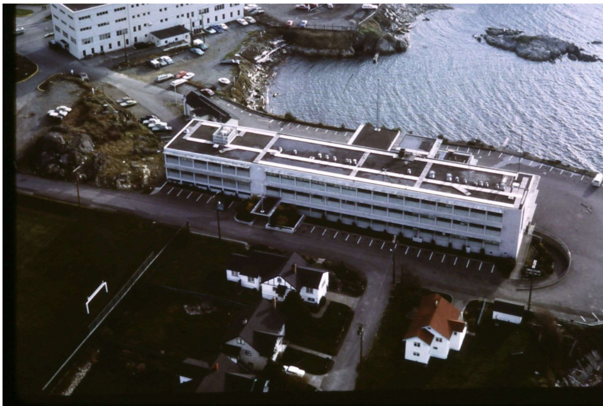
Figure 62: The DREP building is located in the Esquimalt (BC) dockyard area. Photo credit: DRDC.
