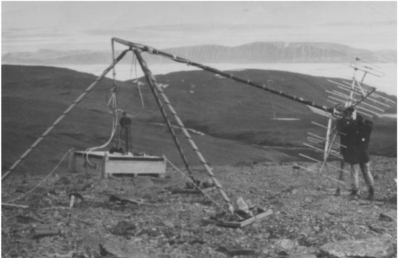
Figure 81: The mast was pivoted on a tripod with the battery box acting as the counterpoise for the antenna. Photo credit: DRDC.
