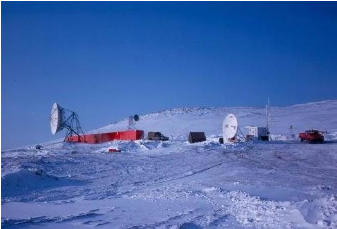
Figure 29: The Skull Point location as seen in April 1982. Upper Paradise is approximately 1000 m behind Skull Point and about 150 m higher. The smaller dish is a 12' (3.6 m) reflector that was installed and used for the original propagation measurements from Skull Point in 1978. Photo credit: Griff Toole. This photo was taken from http://jproc.ca/rrp/alert.html .
