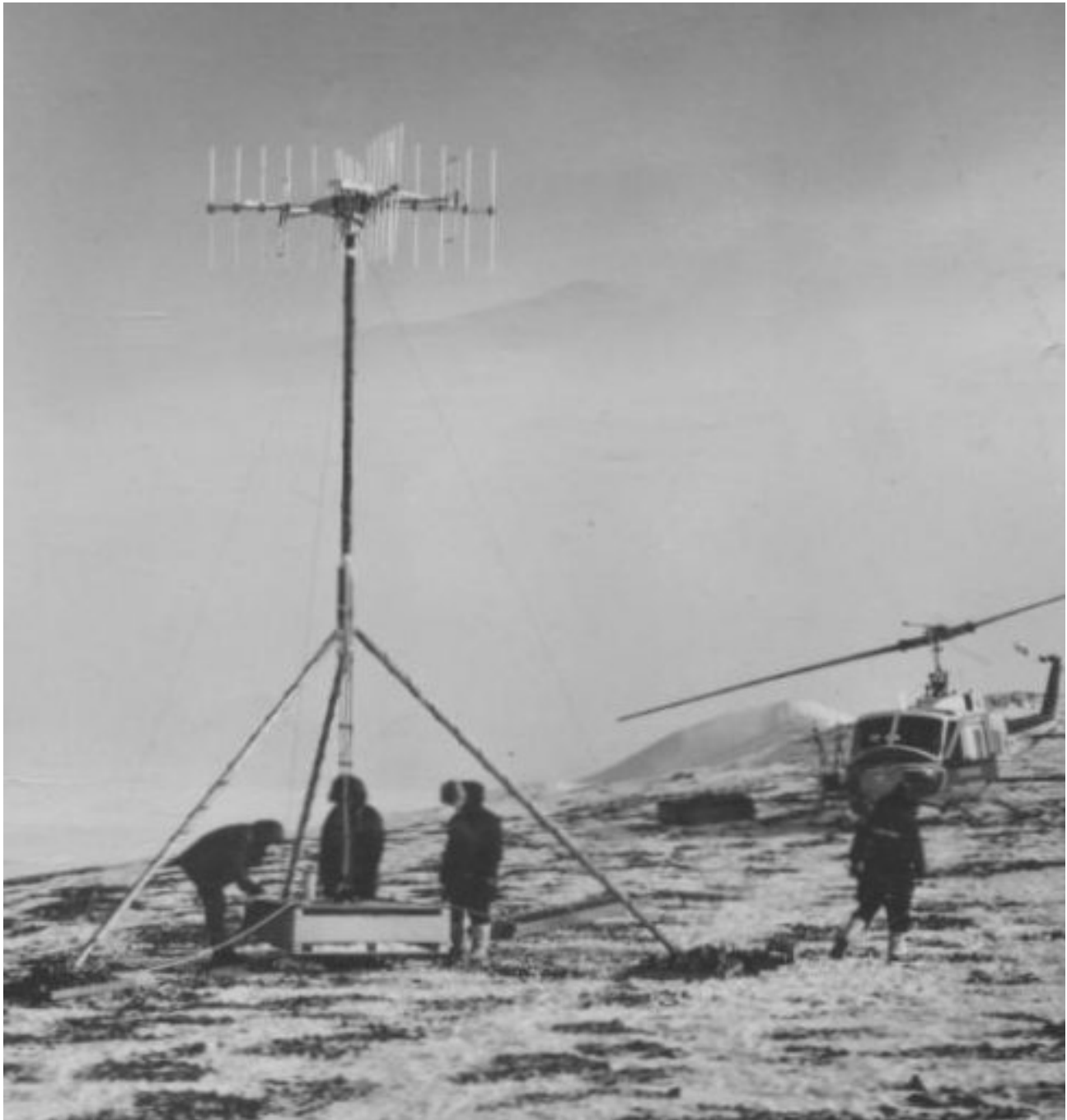
Figure 82: VHF repeater being set up on a high point between Wrangel Bay and Alert. The mast was guyed in place after the battery box had pulled it upright. Photo credit: DRDC.
