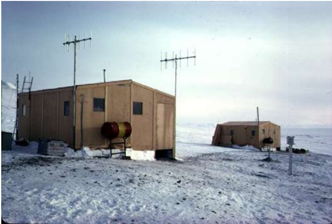
Figure 101: Two of the three buildings at the Fjeldholmen Island shore camp. Photo credit: DRDC.
