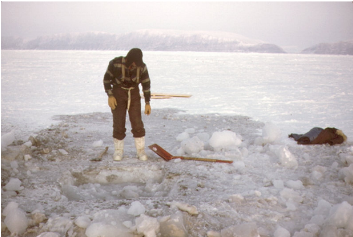
Figure 89: The results of blowing a hole in ice that is about 1.5 m thick. Three one-pound charges were used. Generally, most of the broken ice in the new hole has to be removed by shovel. Photo credit: DRDC.
