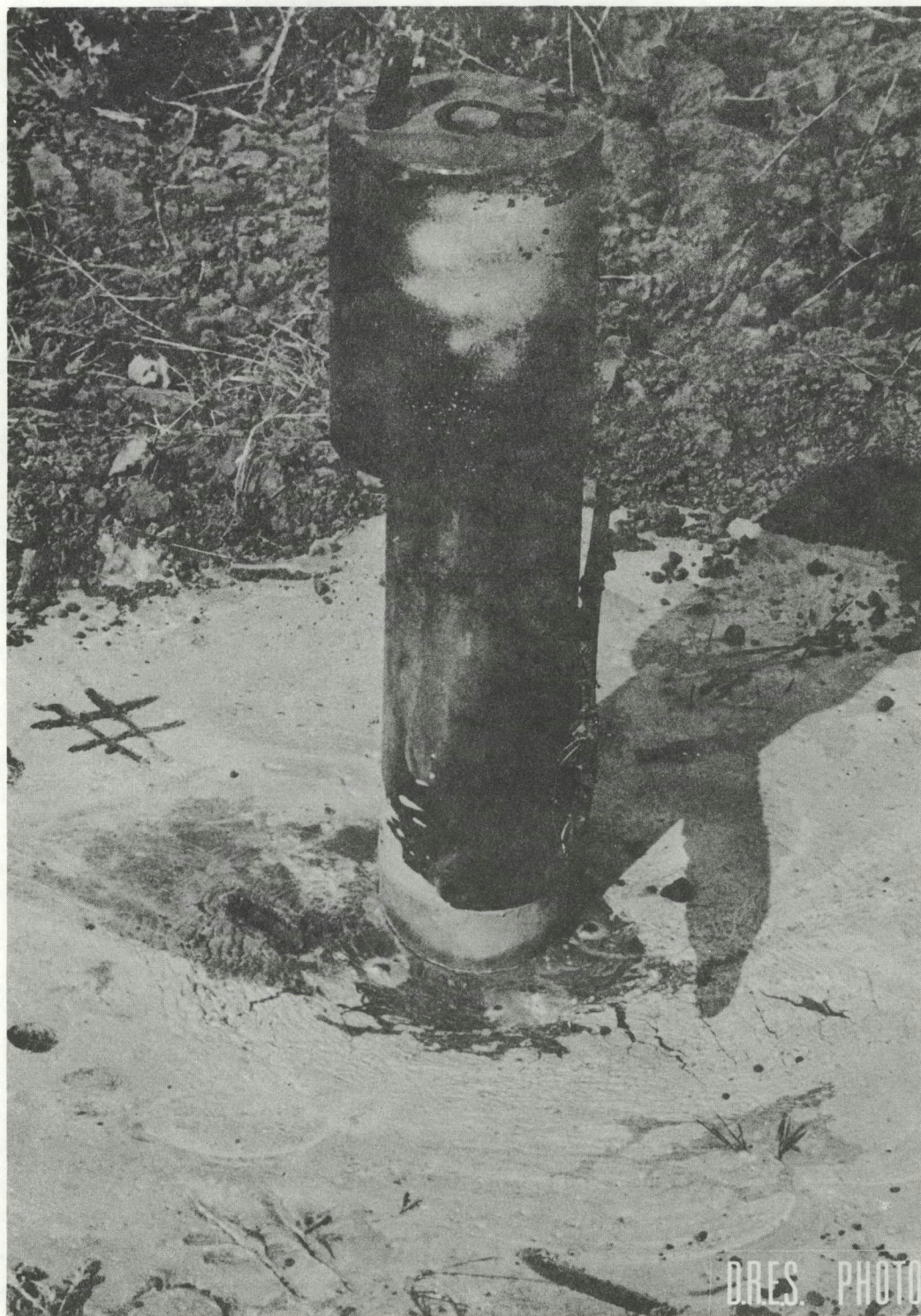
FIG. 5 COMPLETED CASED AUGER HOLE
