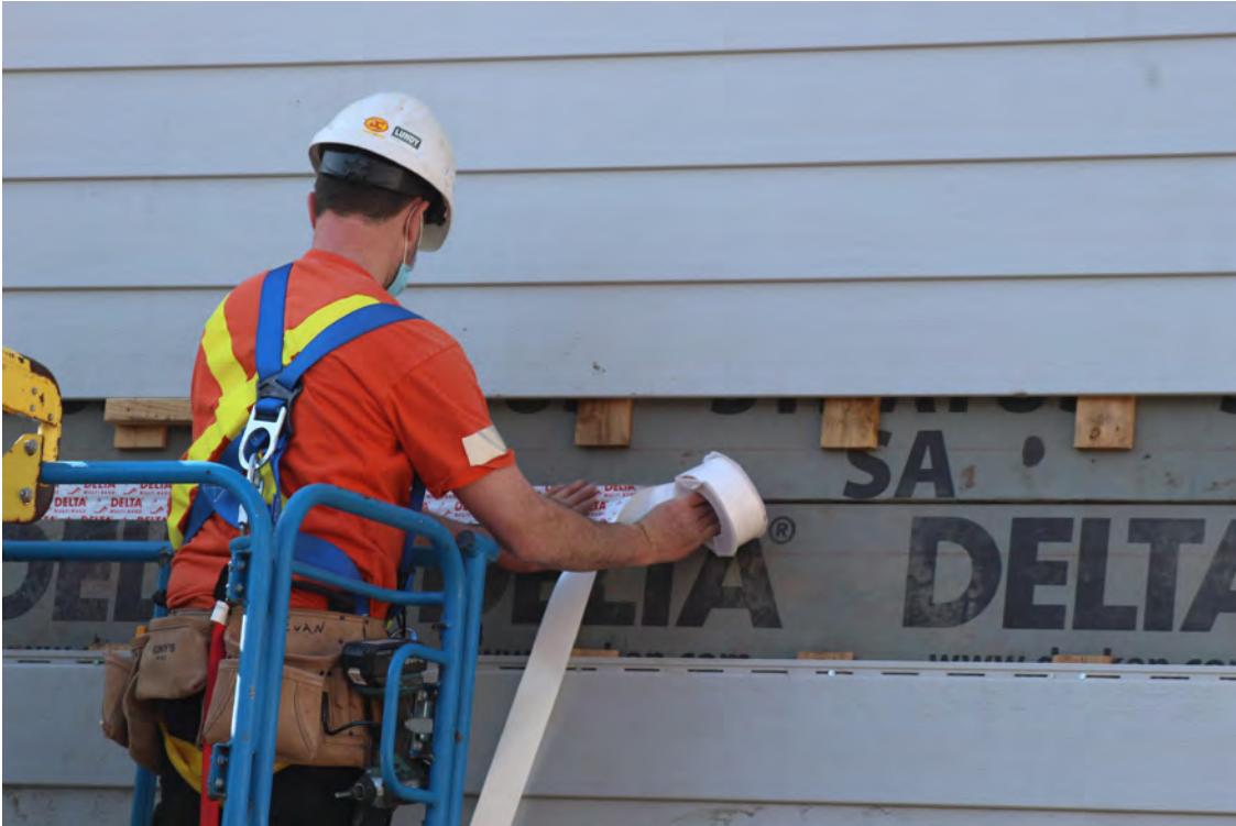
Figure 10-3: Pressure-sensitive acrylic tape being used to seal horizontal panel joint in the field.
