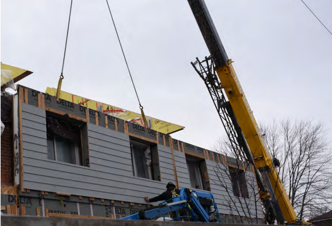
Figure 10-1: A crane proved to be more flexible and faster than a telehandler for hoisting panels for Ottawa Community Housing (OCH)
