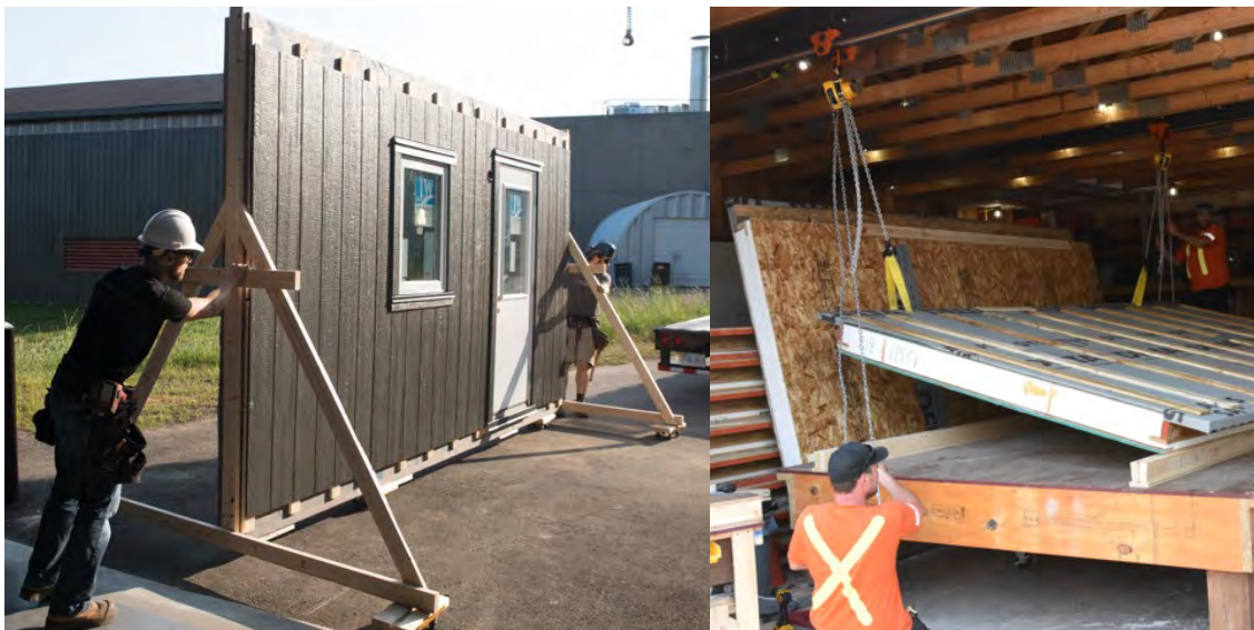
Figure 9-5: (left) Wood outriggers on castors proved to be an affordable and effective way to move panels for the 2017 PEER pilot (right) OCH used hand chain hoists mounted to runners on a steel C-channel that allowed panels to be easily tipped-up and moved within the shop.
