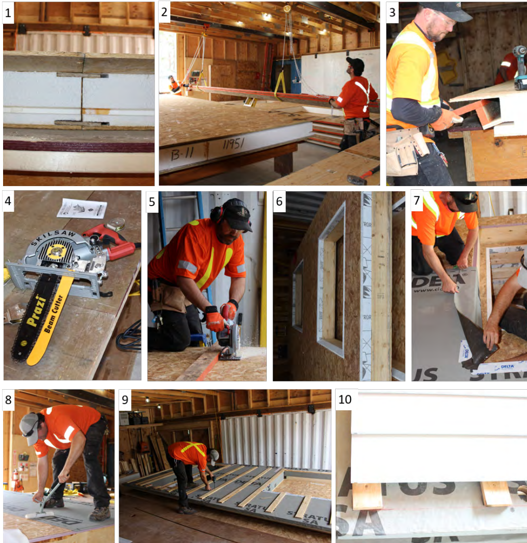
Figure 9-4: SIP fabrication sequence
