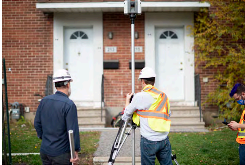
Figure 7-6: Field technicians using a 3D laser (LiDAR) scanner to measure an existing building.
