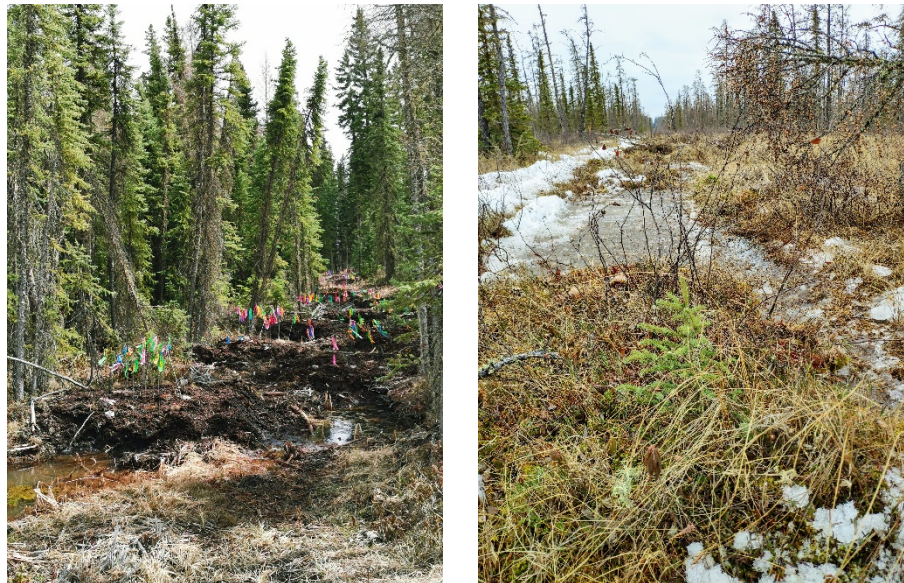
Figure 6. Seismic Line Reclamation Techniques. Left: Mounds created by inverting peat; Right: An upright, transferred hummock on a flat winter road through a treed fen. Courtesy of B. Xu
