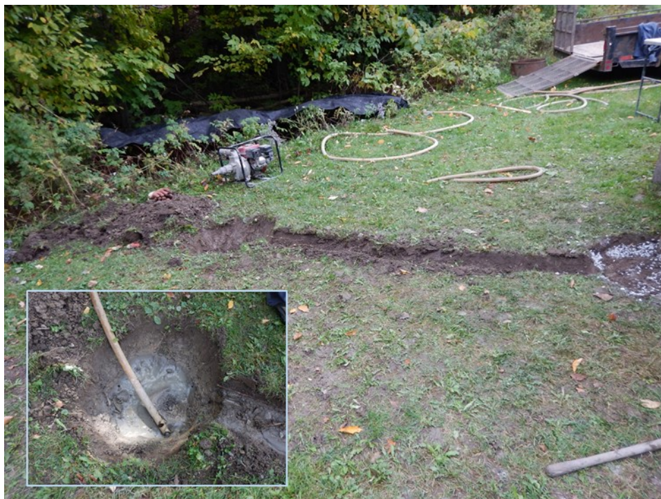
Figure 11. Preparation of drilling sump and sediment bag at site BC16; inset, sump prior to drilling; Photographs by M.J. Hinton, NRCan photo 2022-332, and inset NRCan photo 2022-333
