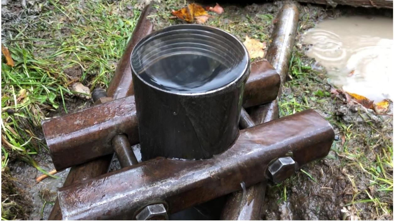
Figure 24. Backflow from the drill casing at a borehole depth of 100' (30.5 m) at site BC16; Photograph by M.J. Hinton, NRCan photo 2022-343
