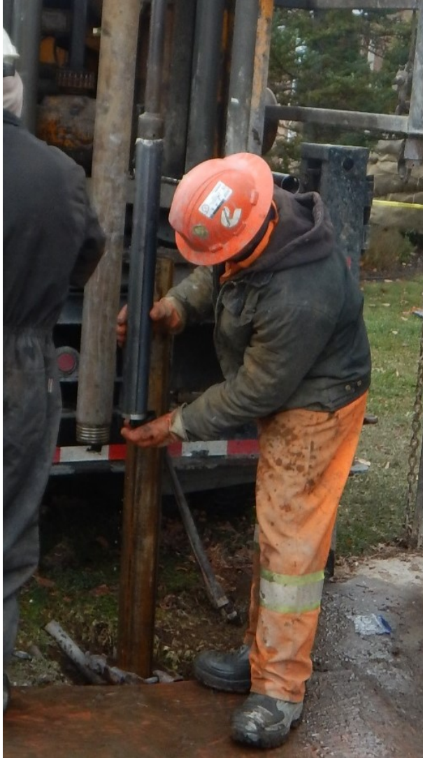
Figure 6. Temporary capping of Shelby tube following sampling with an open tube sampler; Photograph by M.J. Hinton, NRCan photo 2022-327
