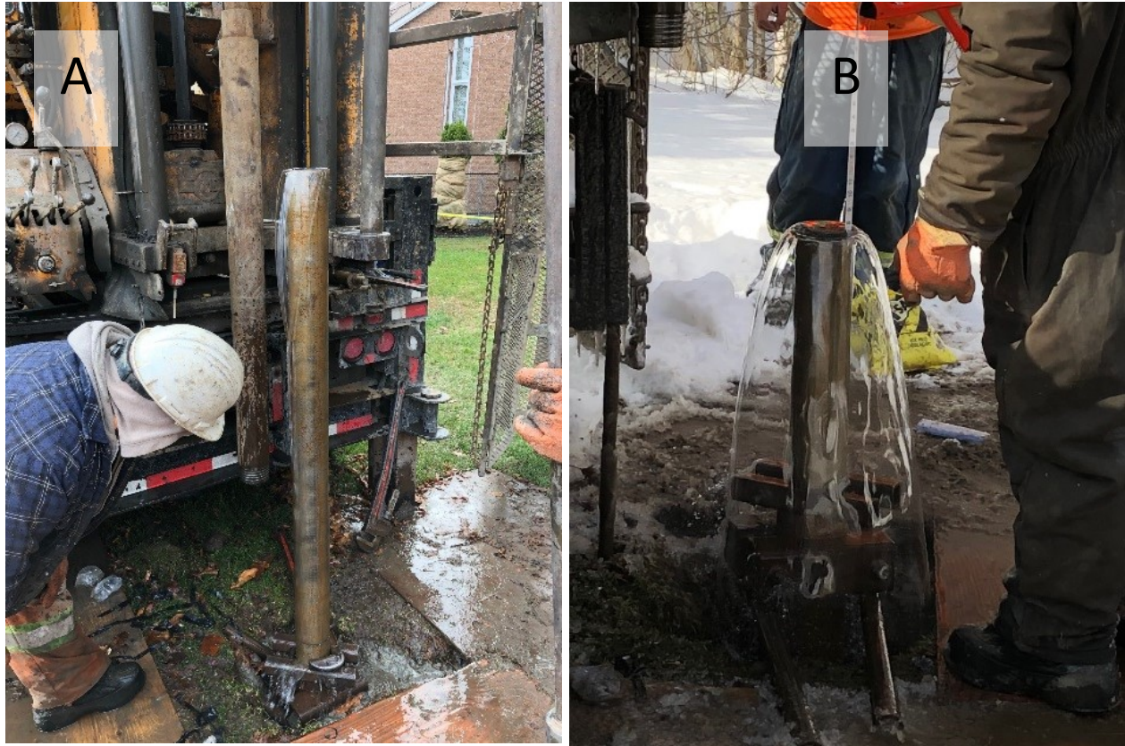
Figure 31. A) Backflow at a borehole depth of 164' (50.0 m) at site VC2; and B) backflow at a borehole depth of 206' (62.8 m); photographs by M.J. Hinton, NRCan photo 2022-347 and 2022-348 respectively
