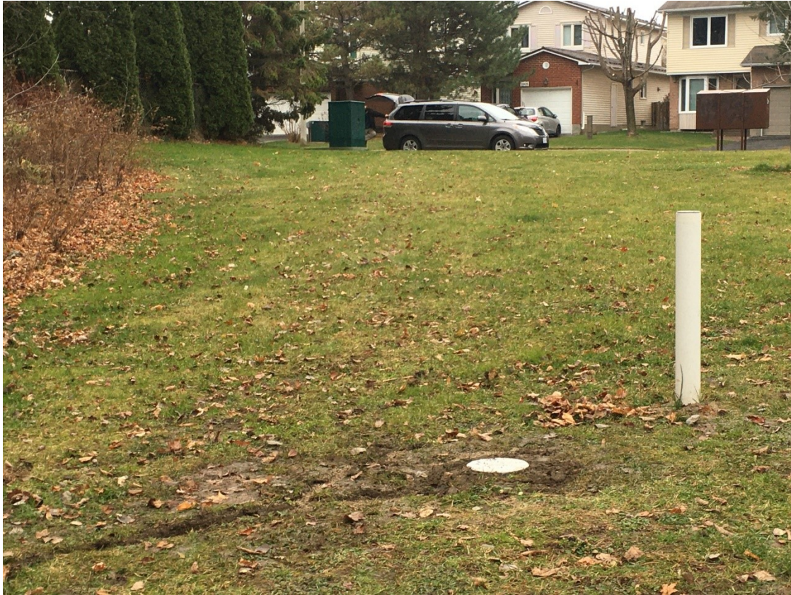
Figure 27. Improved surface drainage for the vibrating wire piezometer, GSC-BC16-p2, installed within the flush mount casing, left; The casing for borehole geophysical logging, GSC-BC16, is on the right. Photograph by S. Alpay, NRCan photo 2022-344
