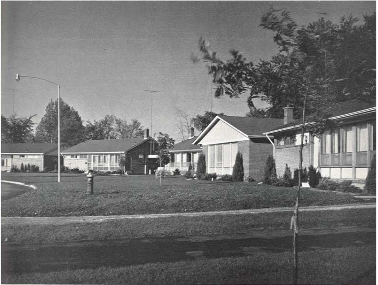
House Grouping, Bayview, Toronto.
