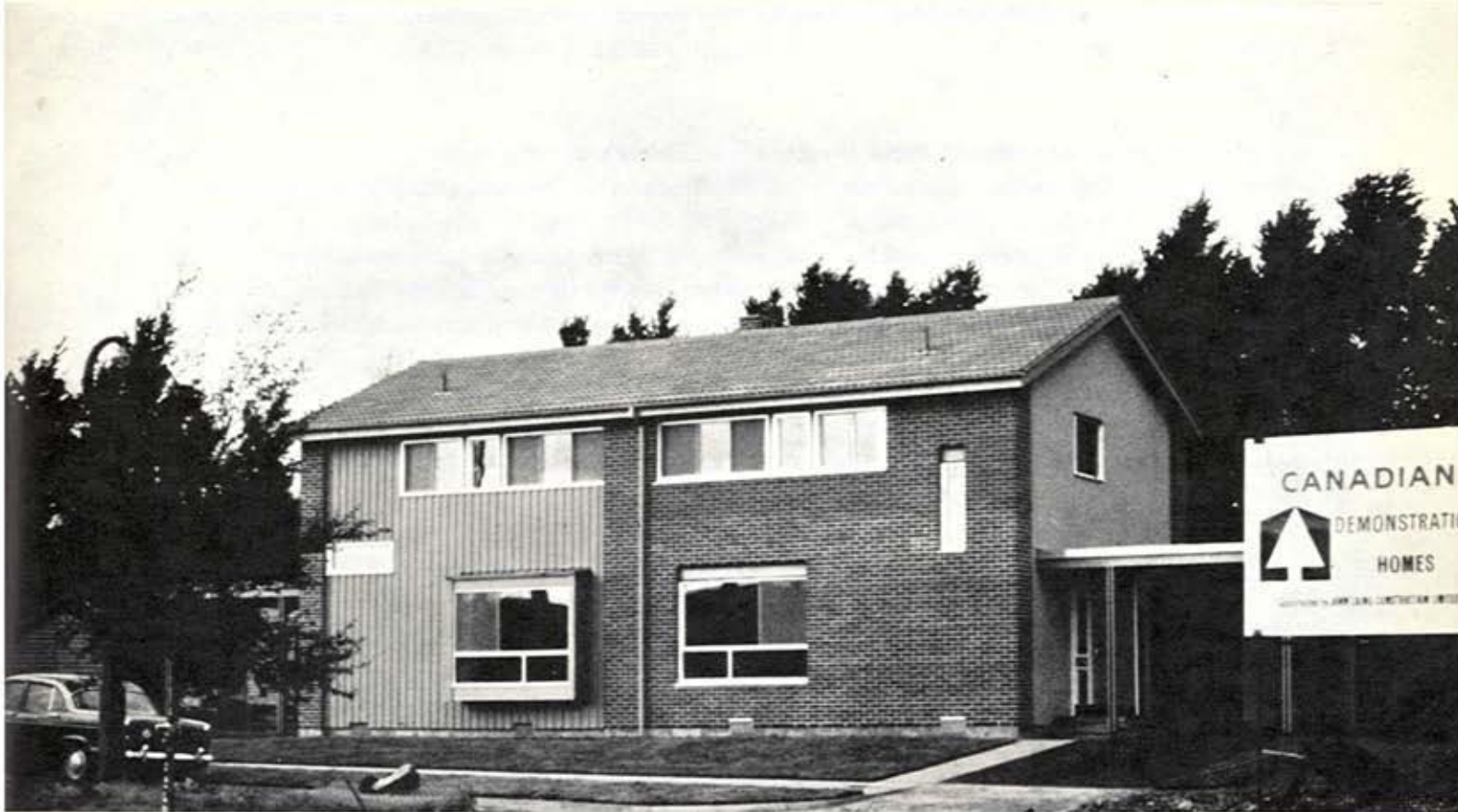
Demonstration houses at Abbots Langley, near London, England, designed and built by the Corporation for the Department of Trade and Commerce, Canada. Three exterior finishes are employed — board and batten, brick and stucco — to illustrate the flexibility of Canadian construction techniques.
