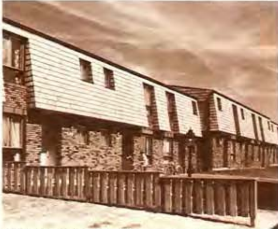
NHA-financed condominium row-housing project, Great Oaks, Sherwood Park, Edmonton, Alta. Designed by D. C. Fairbairn.
