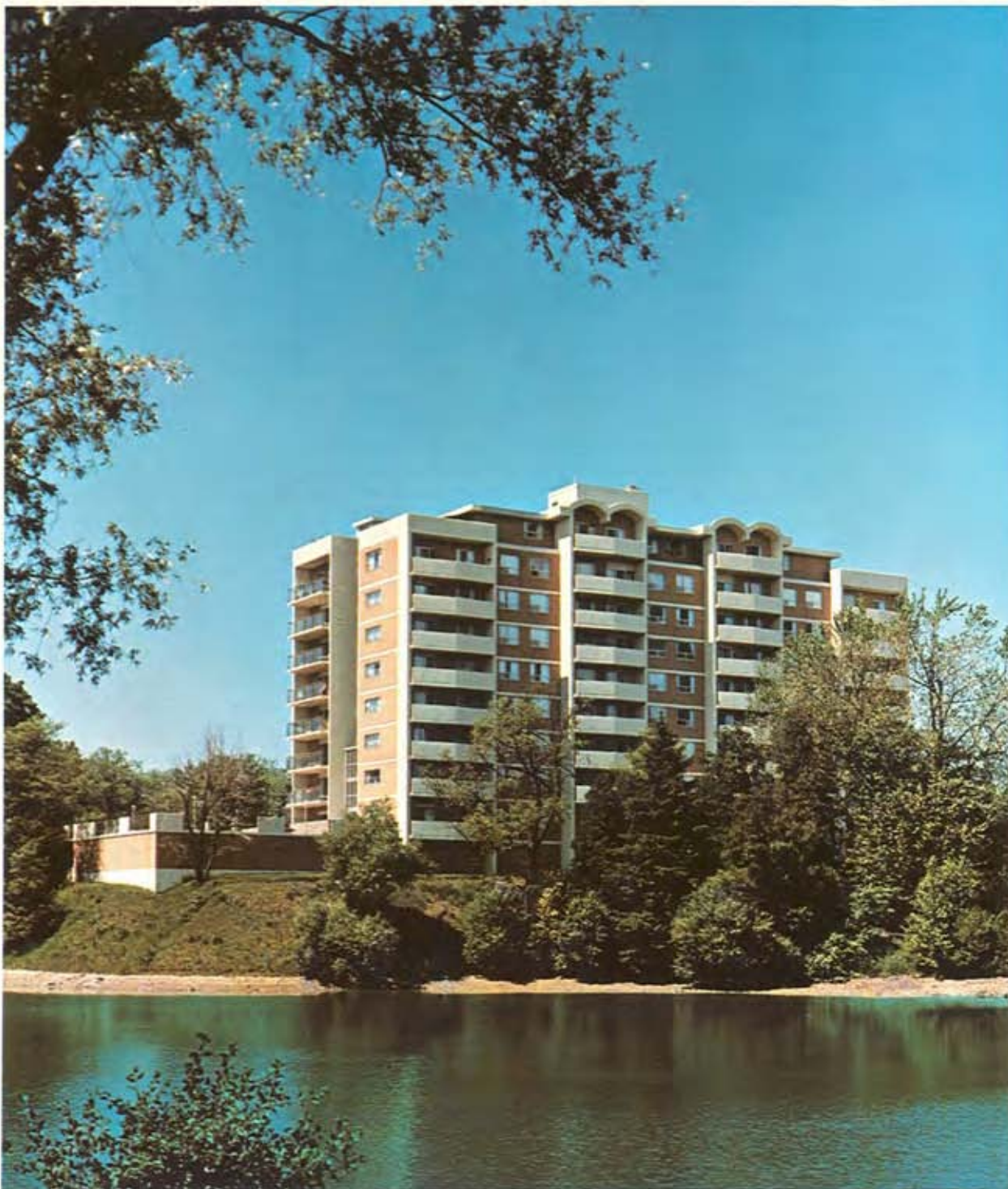
Silver Lake Manor, an NHA-financed apartment building in Waterloo, Ont. Designed by Karl Kruschen.
