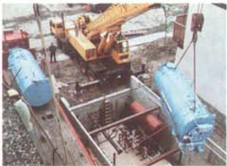
Canada's first low-temperature hot-water heating system is shown being installed for testing in a downtown residential community in Ottawa.
