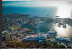
ESQUIMALT GRAVING DOCK Marine Infrastructure Victoria, British Columbia (Public Services and Procurement Canada) Image © Public Services and Procurement Canada
