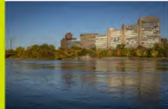
PLACE DU PORTAGE, PHASE III Office Building Gatineau, Quebec (Public Services and Procurement Canada) Image © Public Services and Procurement Canada
