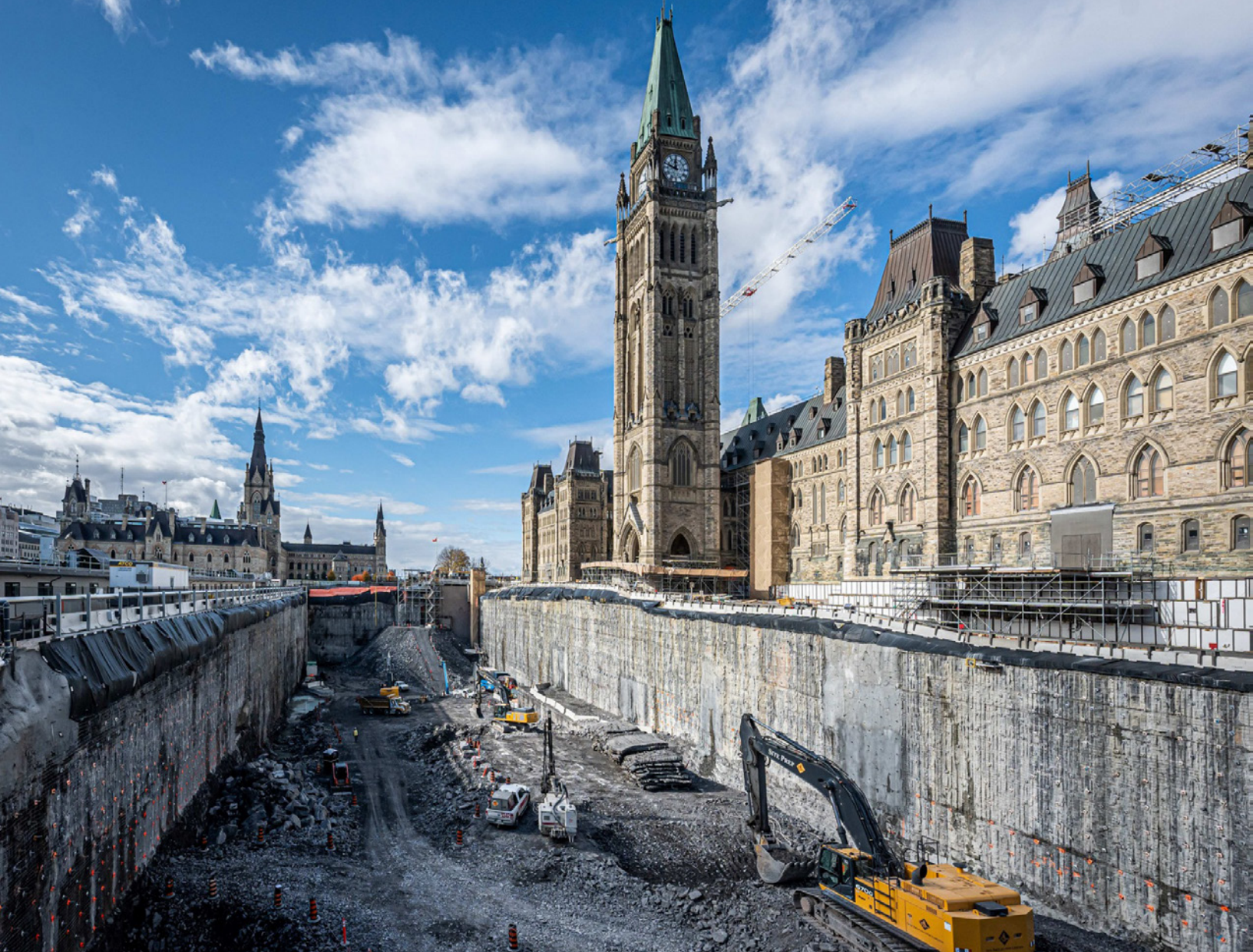
Excavation work at the Centre Block
