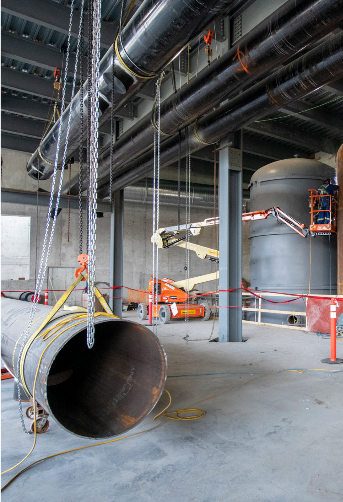
Energy Services Acquisition Program—Tunney's Pasture, Ottawa
