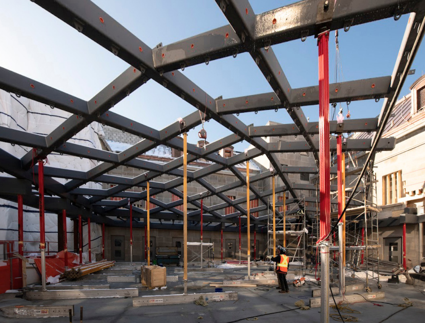
Excavation work at the Centre Block
