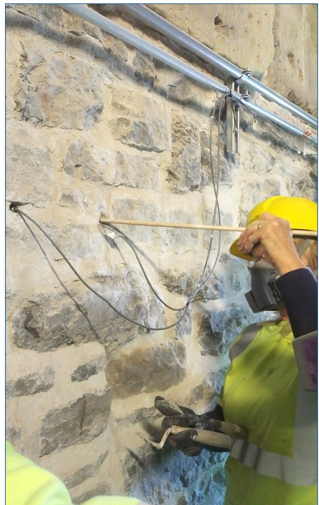
Figure 19: Monitoring sensors being installed in a masonry wall [2]
