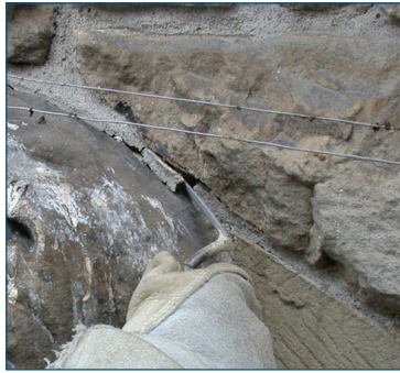
De-bonded Mortar [2]
