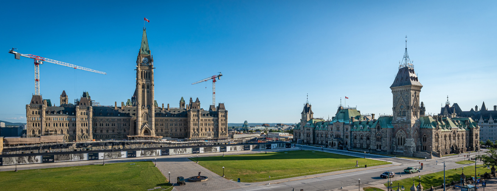
Figure 2: The rehabilitation of Centre Block
