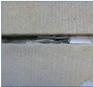
Face-pointing Failure [2]
