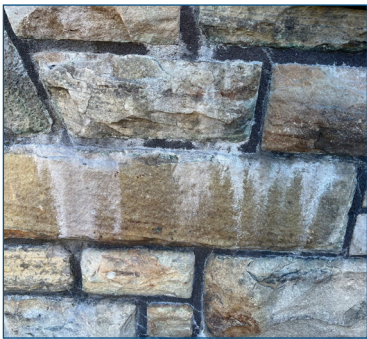
Efflorescence
