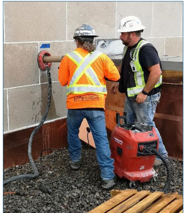
Figure 8: Material sampling being completed at West Memorial Building [4]
