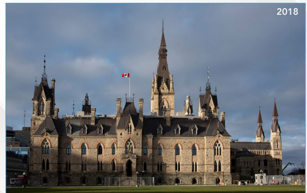
Figure 4: The east elevation of West Block after rehabilitation [1]
