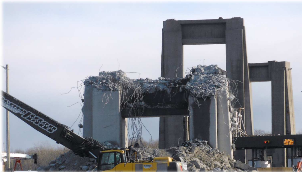
Dismantling the last land pillar next to the “operating in the rubble” toll booth at the Seaway International Bridge in Cornwall.
