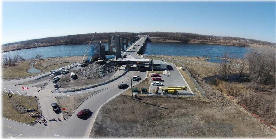
a) Demolition of the high-level North Channel Bridge in Cornwall.
