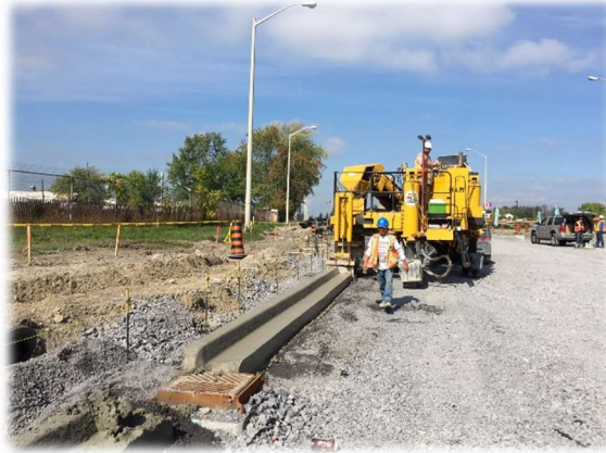
Sewer installation on Brookdale Avenue in Cornwall
