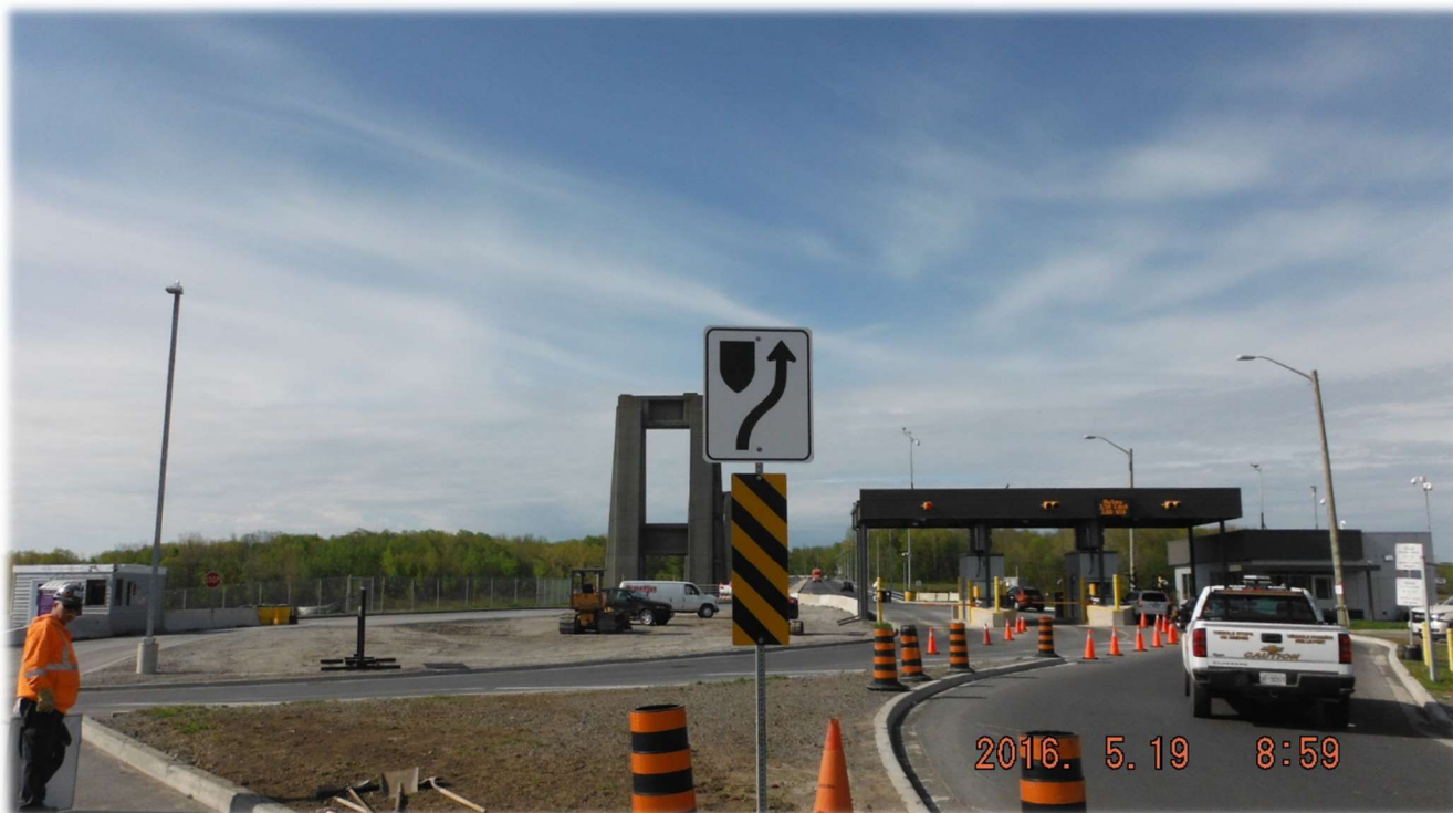
Toll Plaza at the Seaway International Bridge with remaining piers from the old North Channel Bridge
