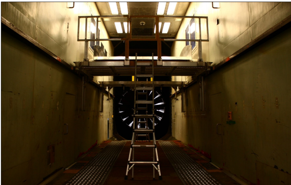
Photo 2.2: Inside View of the NRC Wind Tunnel Test Section
