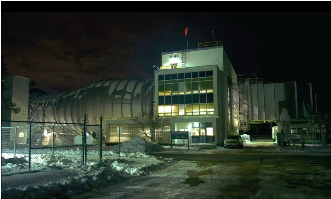
Photo 2.1: Outside View of the NRC Wind Tunnel Facility
