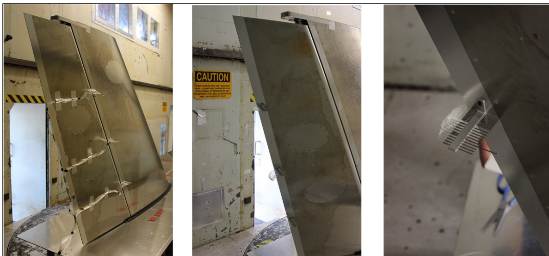
Photo 5.6: Additional Photos of Boundary Layer Rake Installation
