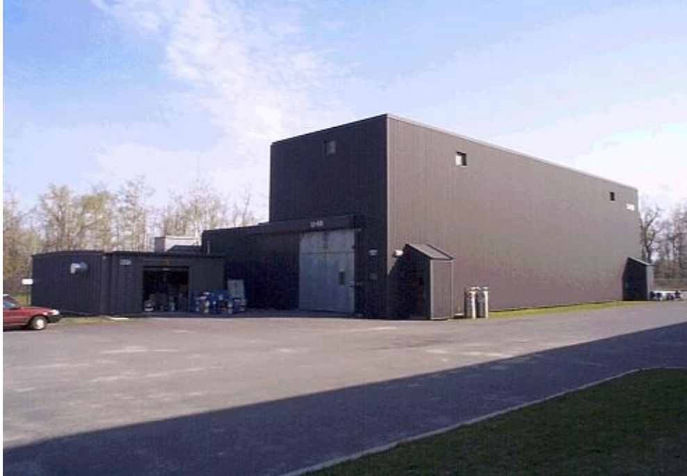
Photo 2.9: Outdoor View of National Research Council Canada Facility
