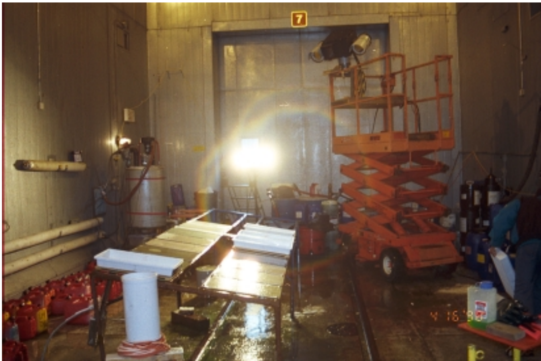
Photo 2.4: Inside View of Small End of NRC Facility
