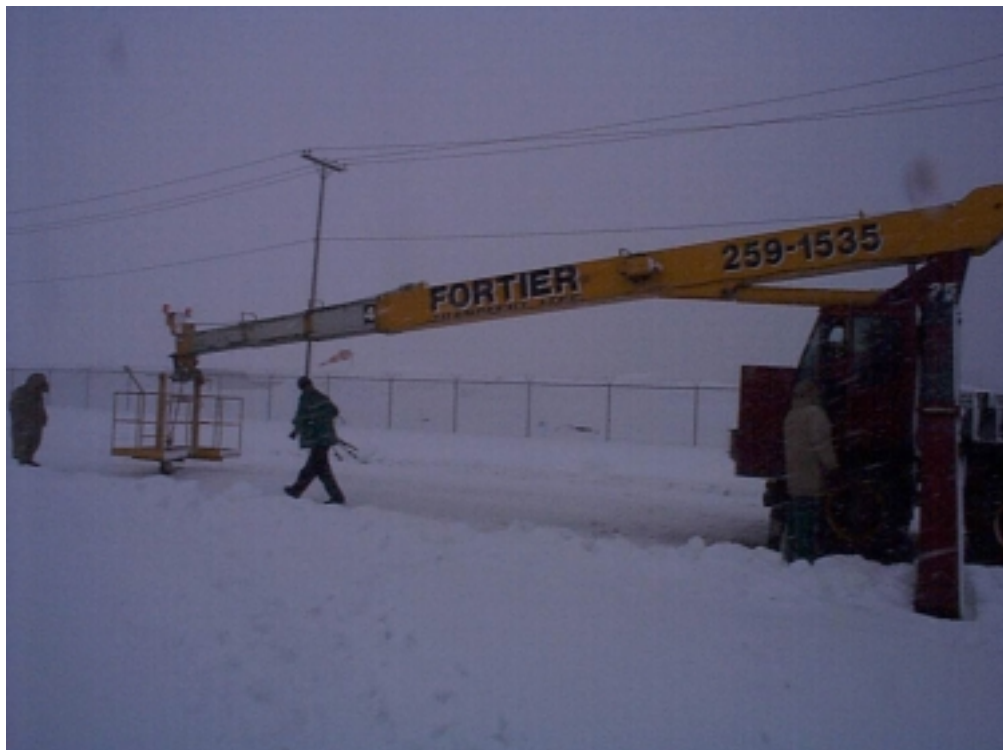
Photo 2.2: Personnel Basket Installed on Mast
