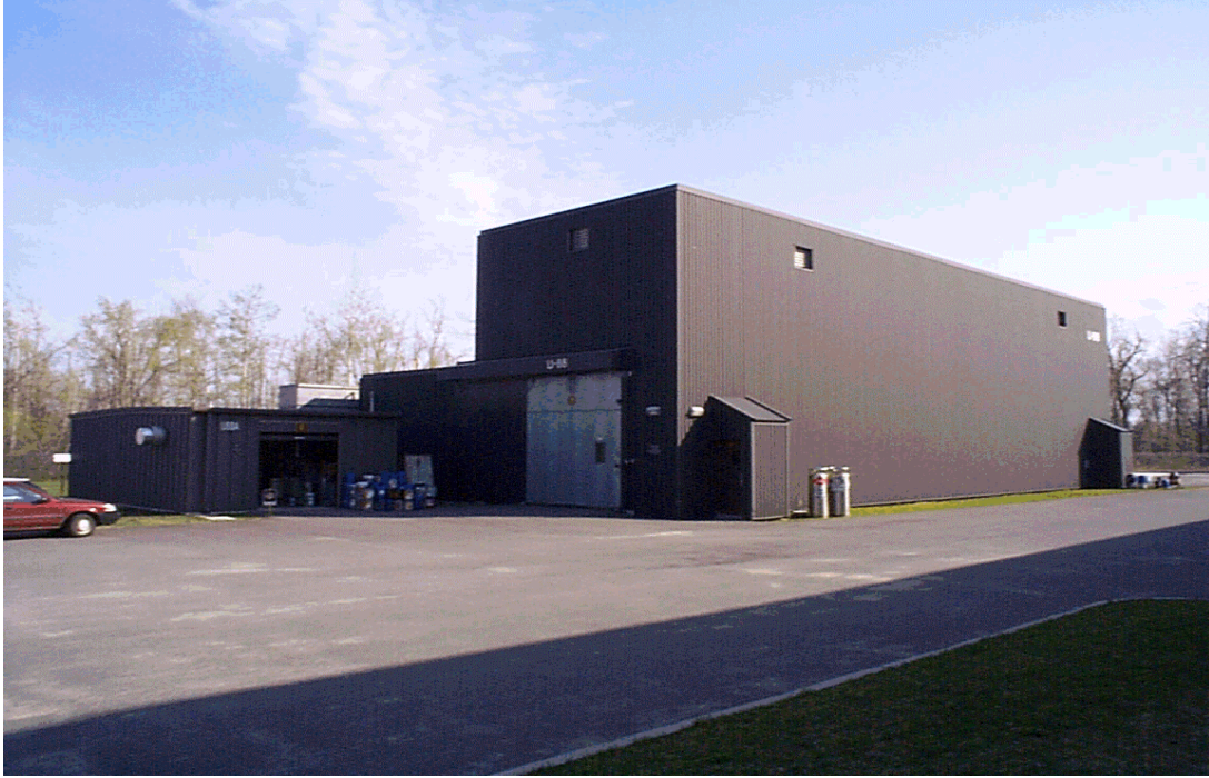
Photo 2.11: Outdoor View of National Research Council Canada Climatic Engineering Facility
