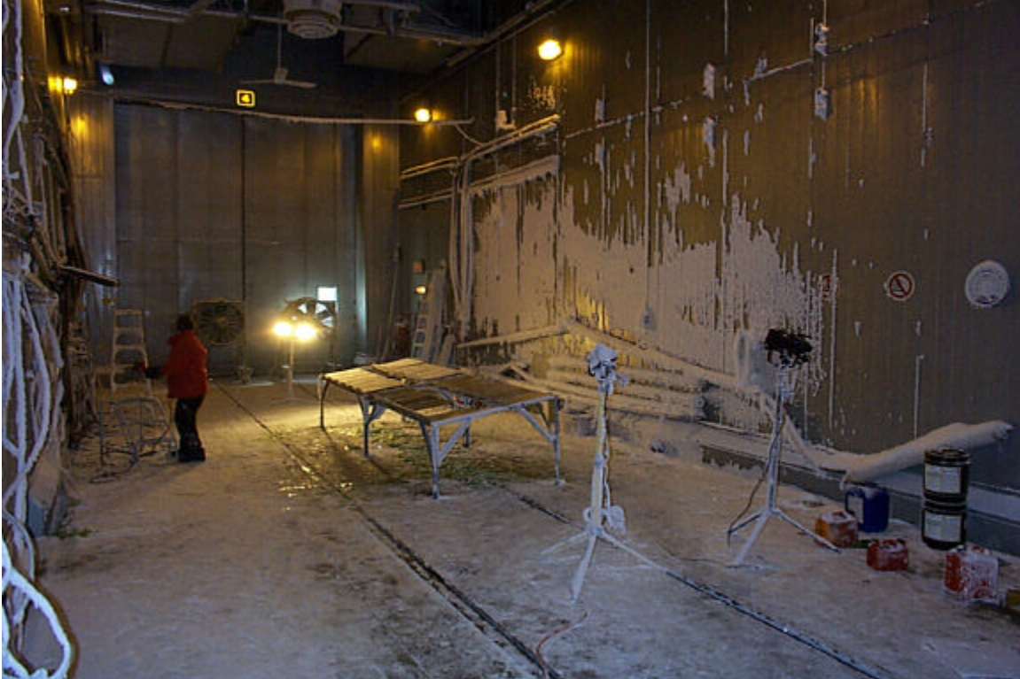
Photo 3.3 Inside View of Large End of Climatic Engineering Facility
