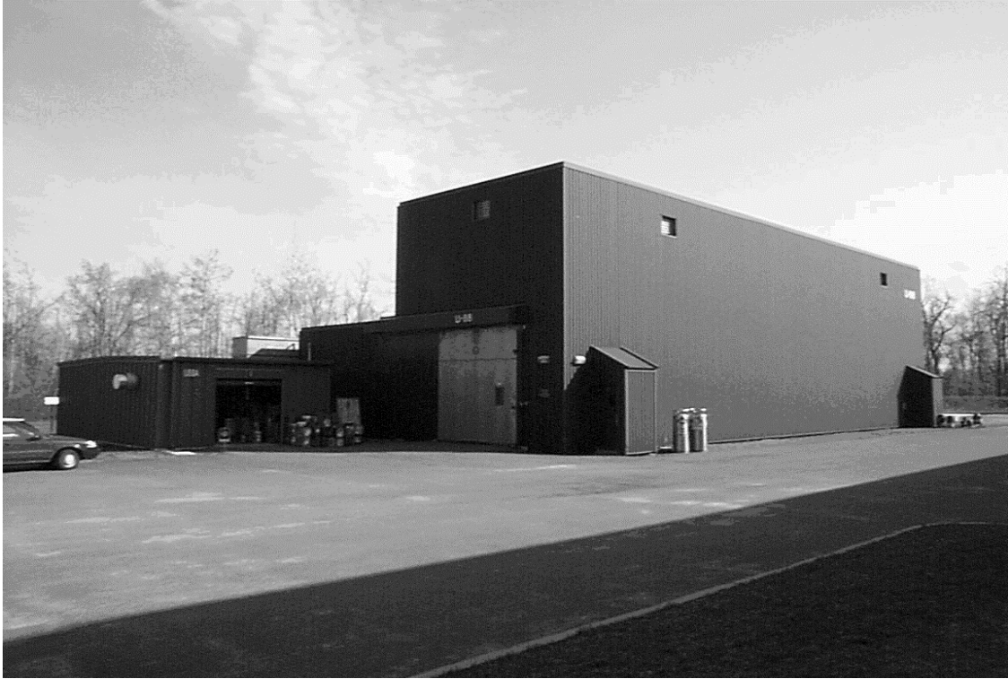
Photo 2.1 Outside View of National Research Council Climatic Engineering Facility
