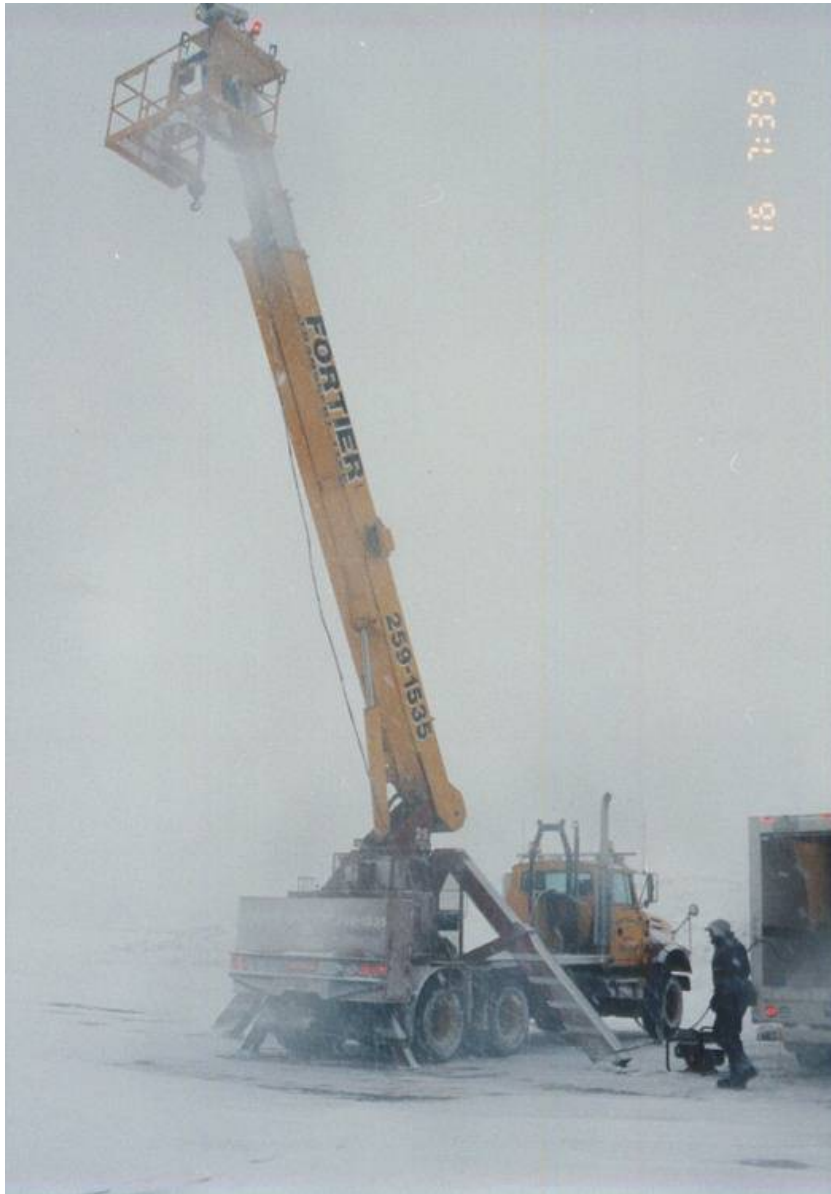
Photo 2.1 Mobile Crane with Sensor Installed
