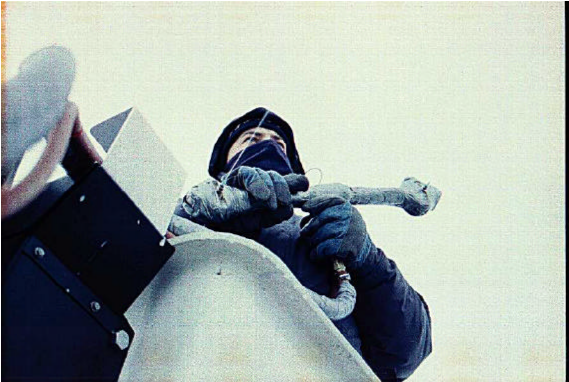
Photo 2.11 Applying Water Spray from Bucket
