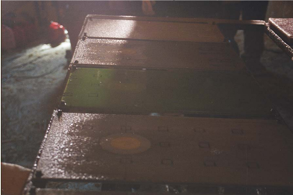
Photo C28.1 - After Pouring, t = 0 min
