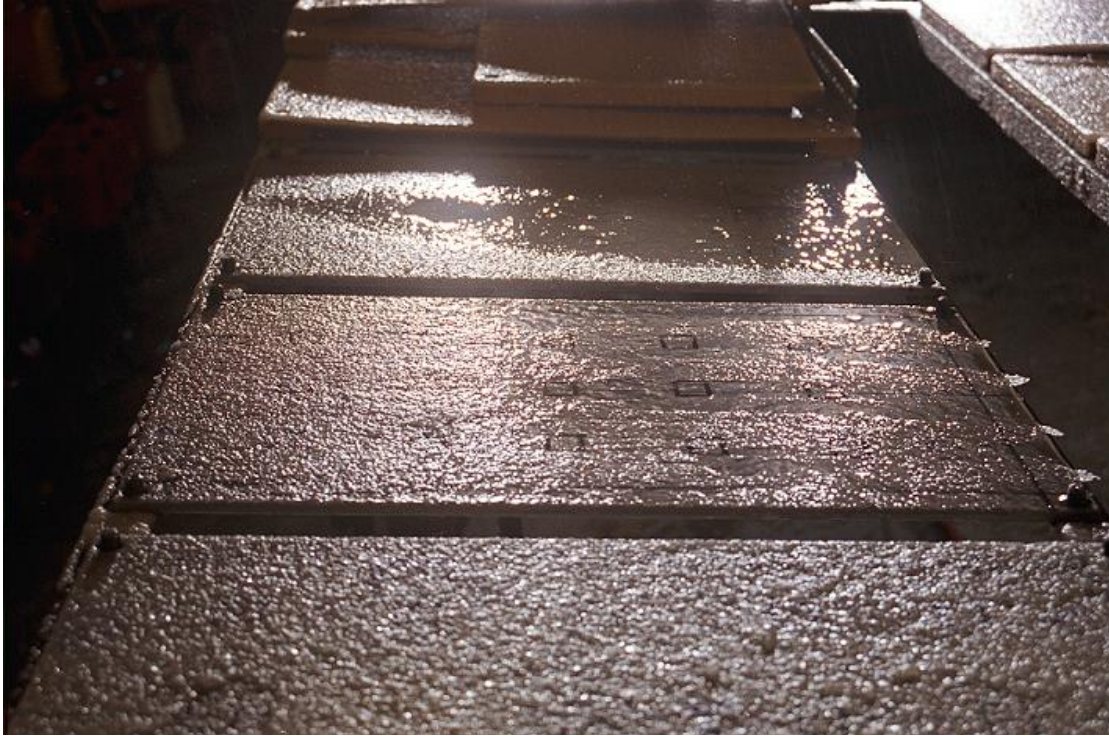
Photo 3.11 Drainage Channels and Fingers
