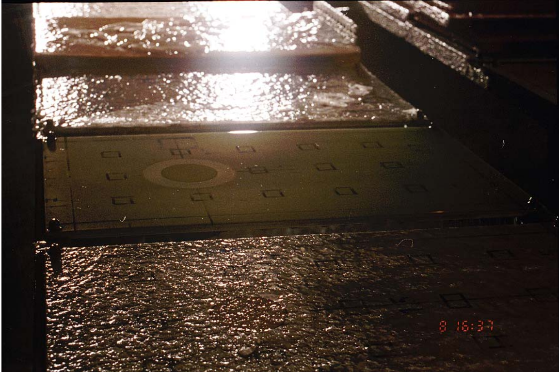
Photo C11.1 - After Pouring, t = 0 min
