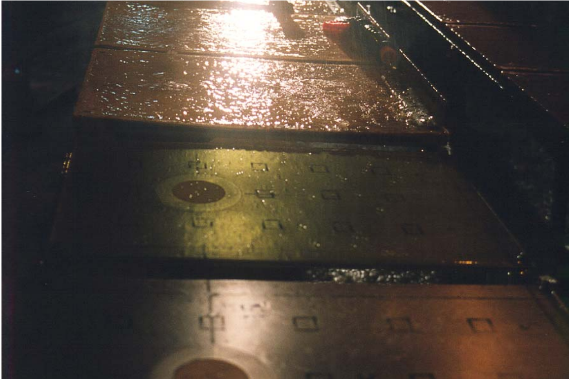
Photo C19.1 - After Pouring, t = 0 min
