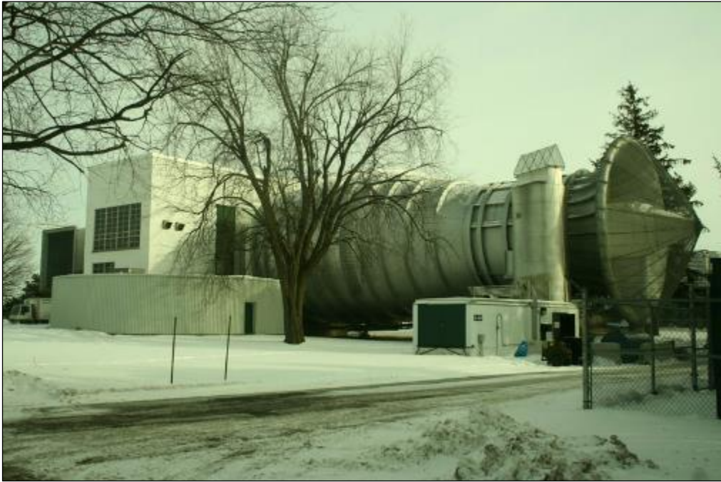
Photo 2.1: Outside View of NRC Wind Tunnel Facility
