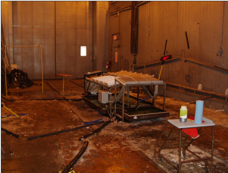
Photo 2.2: Inside View of NRC Climate Engineering Facility
