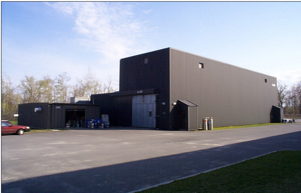
Photo 2.4: Outdoor View of NRC Facility
