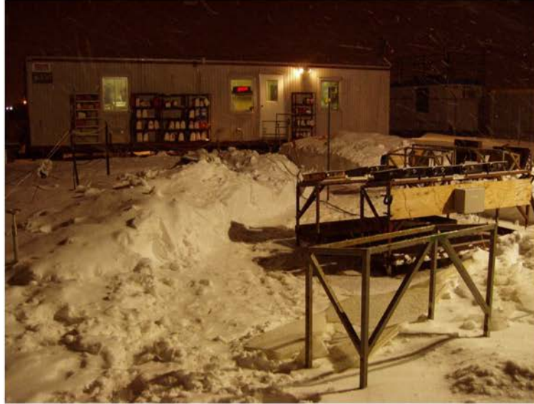
Photo 2.1: APS Test Site - View from Test Pad
