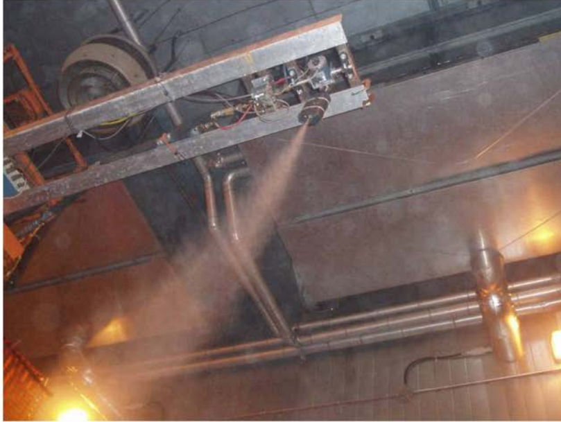
Photo 3.7: Sprayer Assembly in Use
