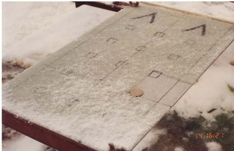
Photo 2: Snow Bridging Failure
