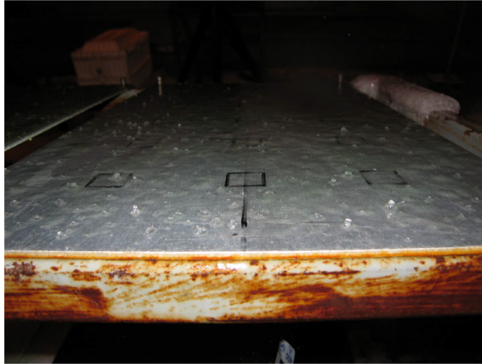
Photo 5.15: Test #RIP 5 – Condition at 20 Minutes
