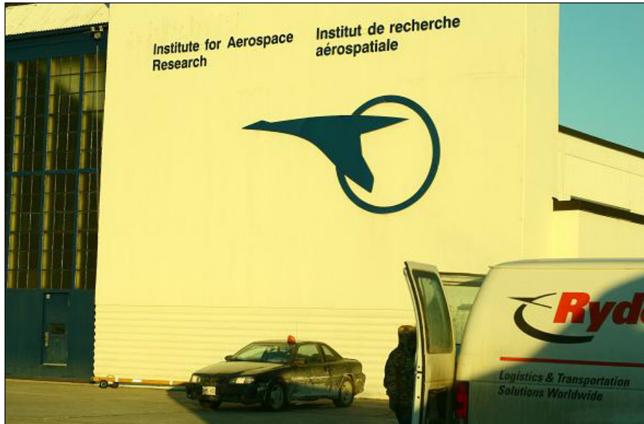
Photo 2.13: NRC YOW Institute for Aerospace Research Hangar
