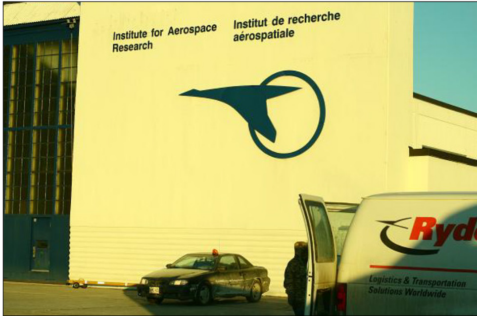
Photo 2.1: NRC YOW Institute for Aerospace Research Hangar
