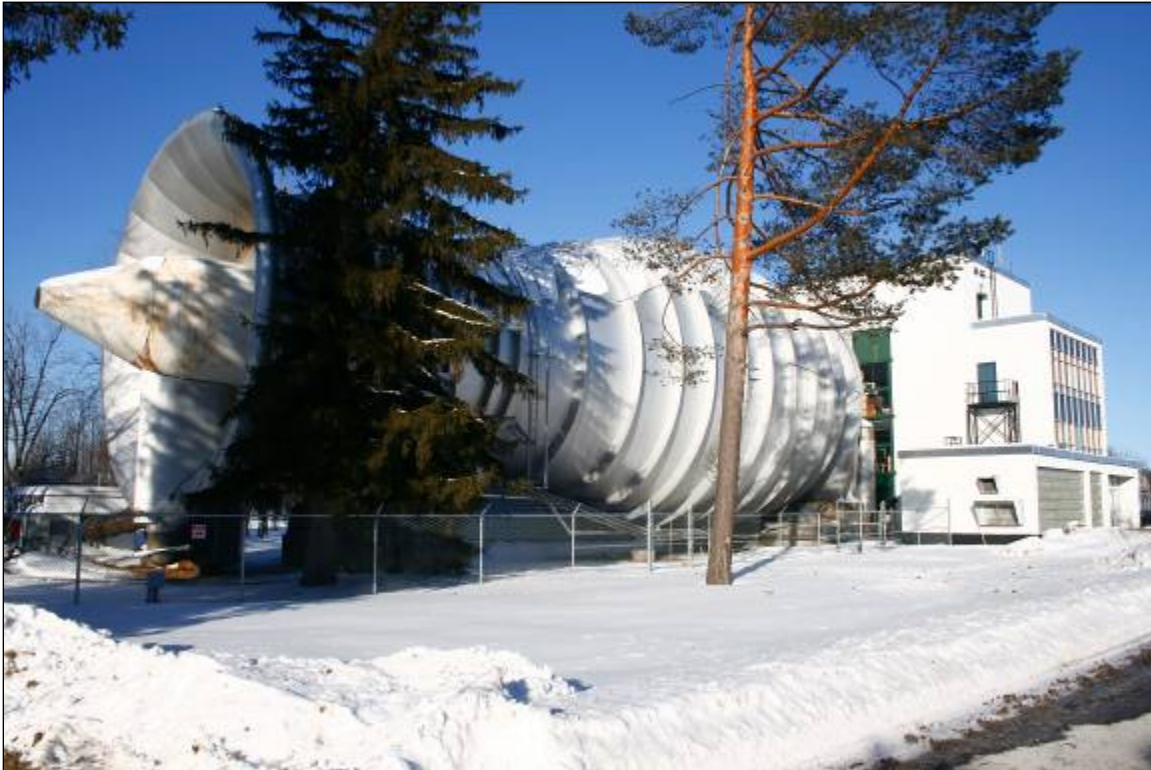
Photo 2.1: Outside View of NRC Wind Tunnel Facility
