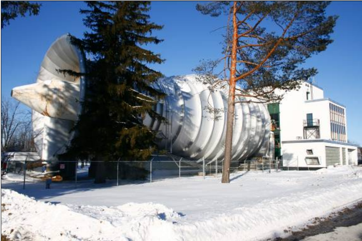
Photo 2.1: Outside View of NRC Wind Tunnel Facility
