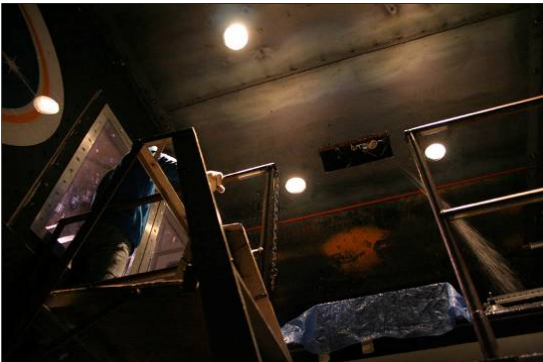
Photo 2.8: Ceiling-Mounted Freezing Rain Sprayer
