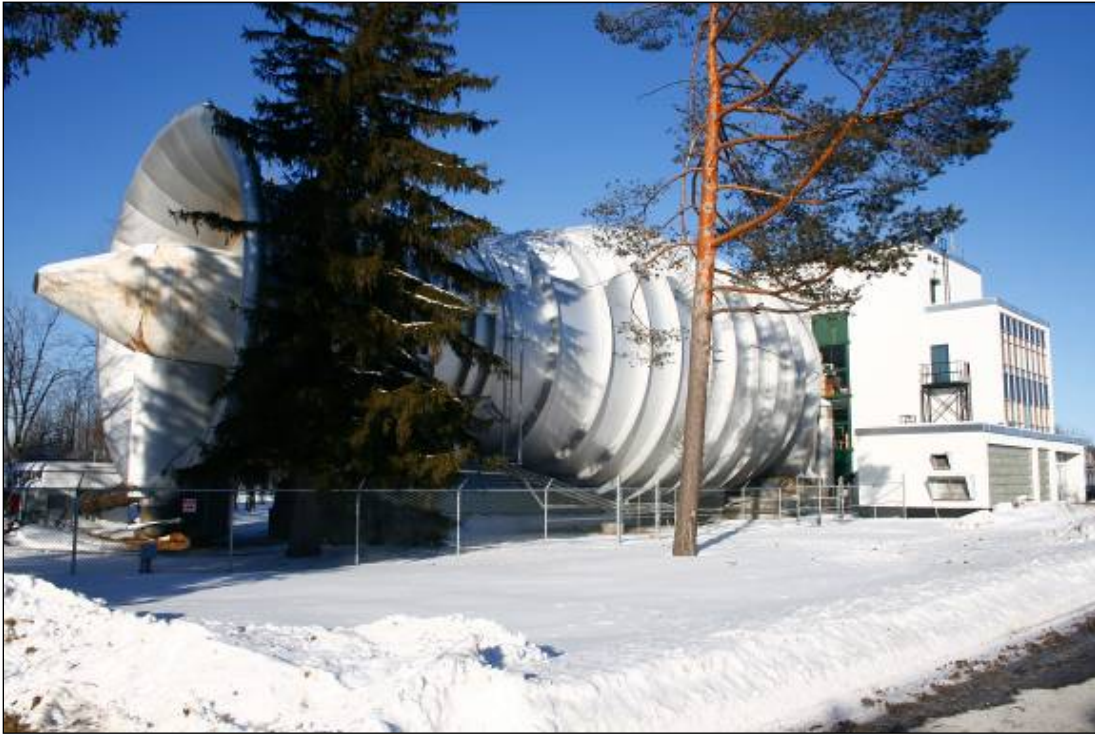
Photo 2.1: Outside View of NRC Wind Tunnel Facility
