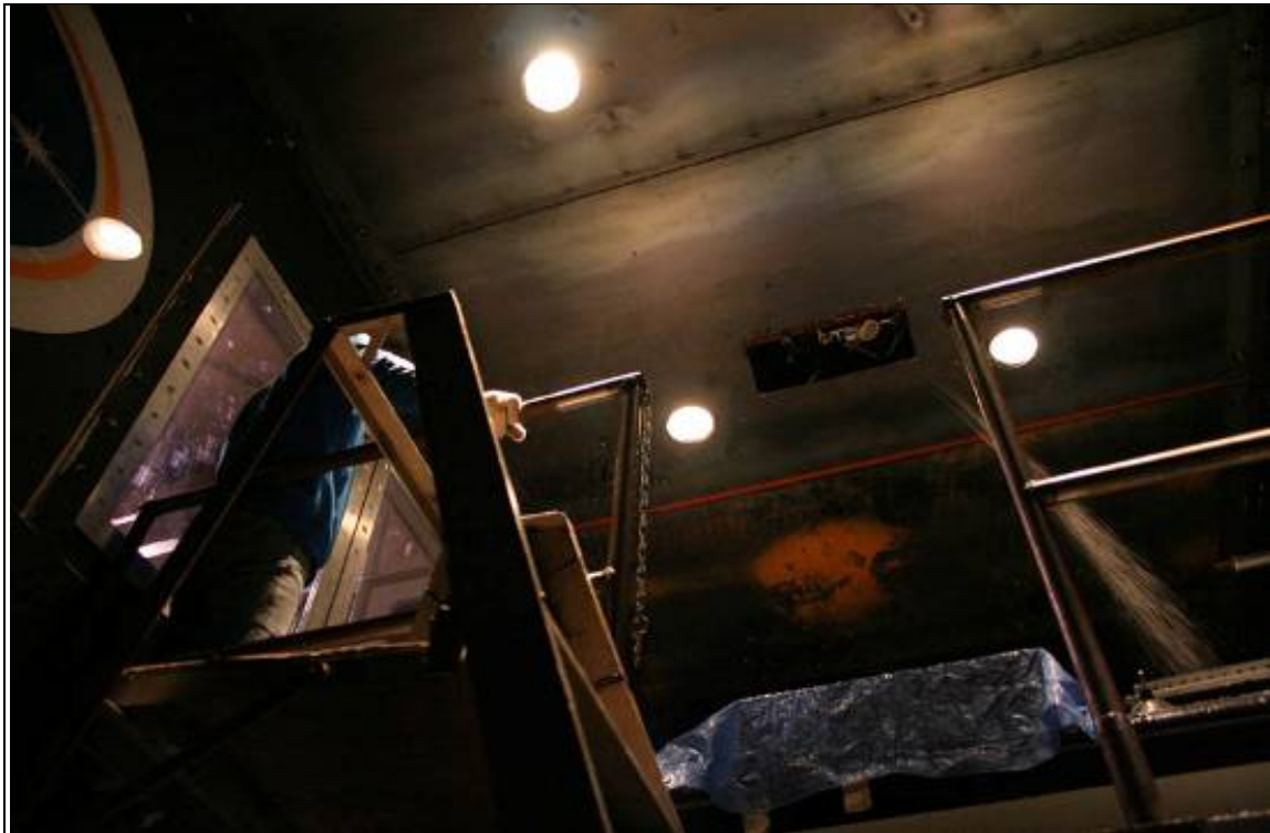
Photo 2.8: Ceiling-Mounted Freezing Rain Sprayer
