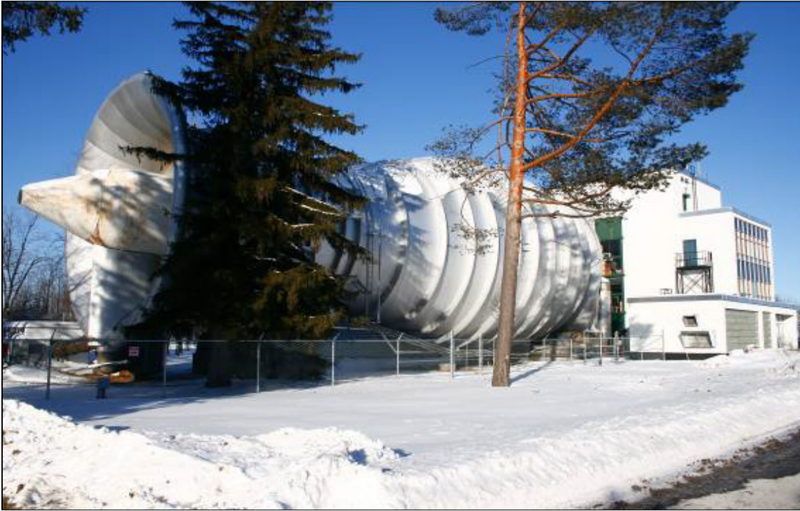
Photo 2.1: Outside View of NRC Wind Tunnel Facility
