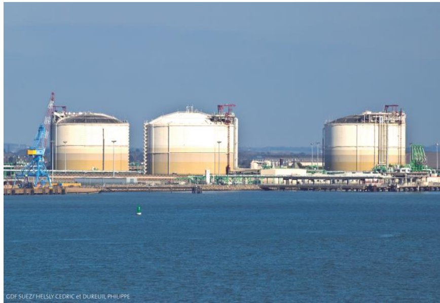
Figure 9: Bulk LNG Storage Tanks (Courtesy of Gaztransport & Technigaz (GTT))
