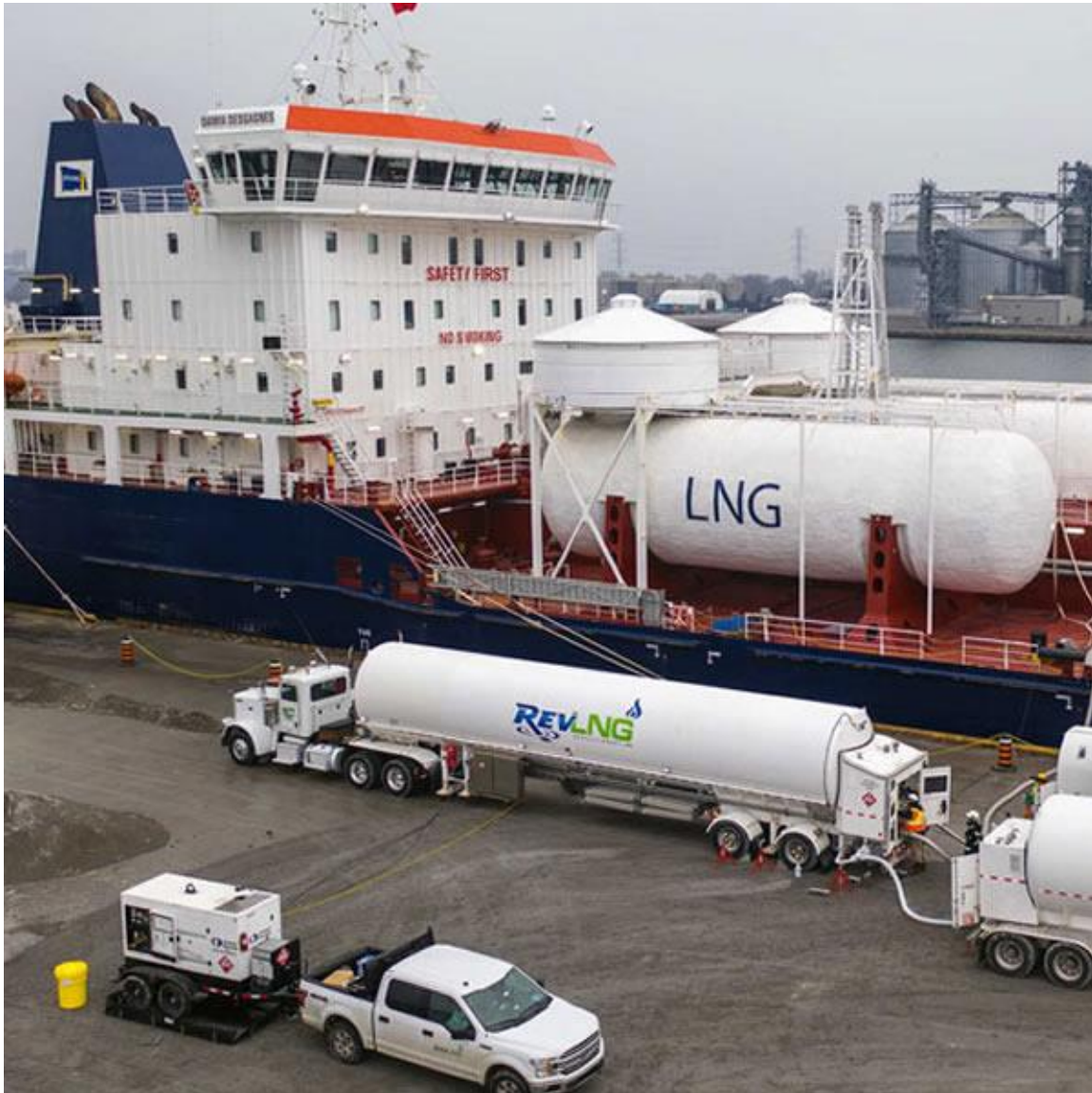
Figure 91: REV LNG truck to ship bunkering in Hamilton, Ont.
