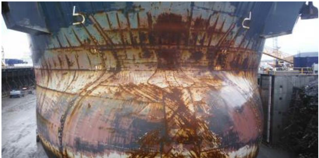
Figure 3: The vessel’s bow before upgrades 3
