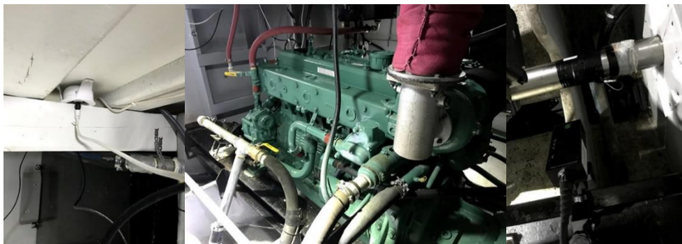
Figure A - 44 Boat Engine Room and Installed Torque and Speed Sensors
