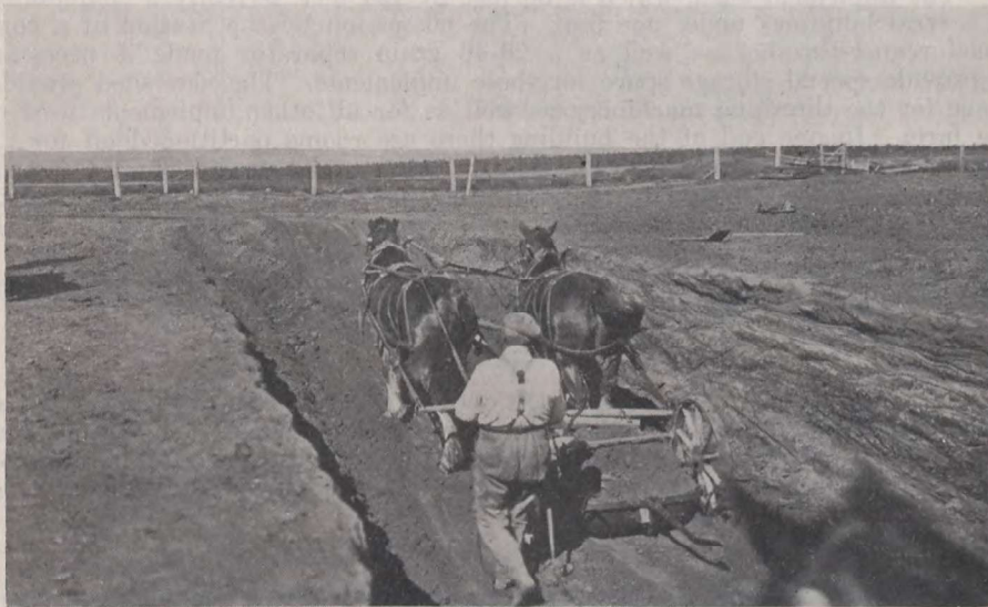
Excavating trench silo with wheel scraper.
