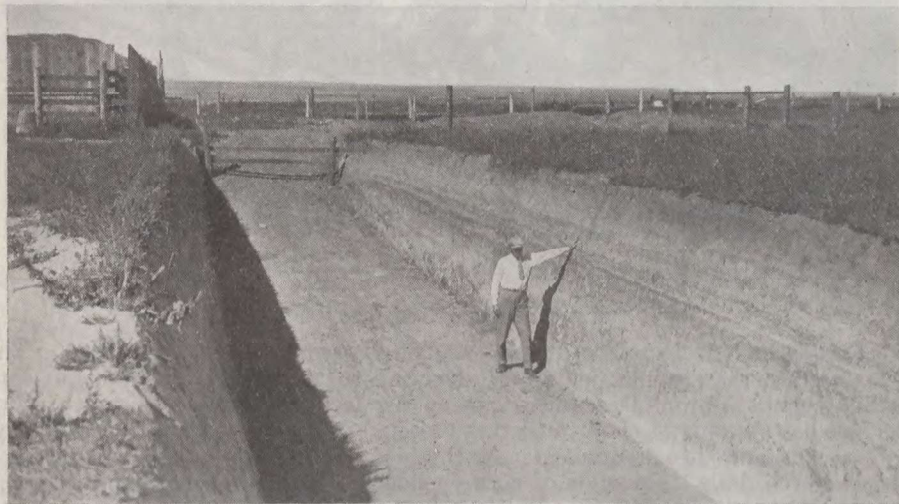
Trench silo ready for filling.
