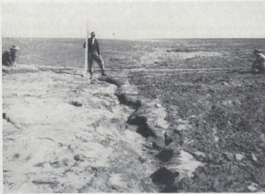
FIG. 27.—Water erosion damage. Note the shallow top soil and the exposed clay and stone. The top line indicates the original surface.
