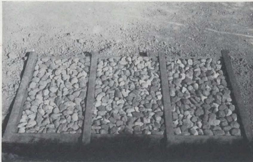
FIG. 24.—Sand, gravel, and rock filter in place at bottom of a dugout. Filtering water for the domestic water supply in the house.
