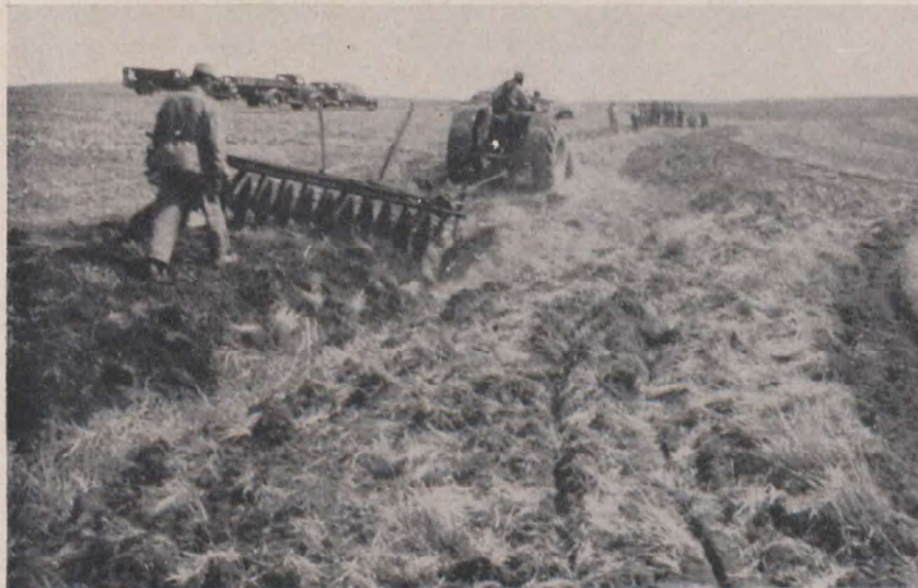
FIG. 8 Constructing a grassed waterway with a one-way disk.
